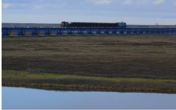
Figure 11. Cargo train on the bridge over the Yuribei River floodplain traveling to the Bovanenkovo gas field. (Photo: T. Kumpula, July 7, 2010)
