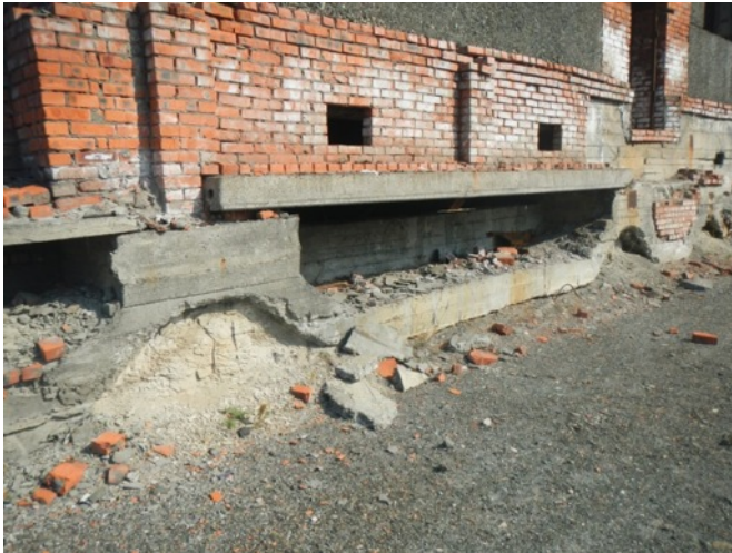
Figure 30. Profile of typical surface foundation used on permafrost with high ice content (top) and example of building with such foundation in Oganer (bottom).
