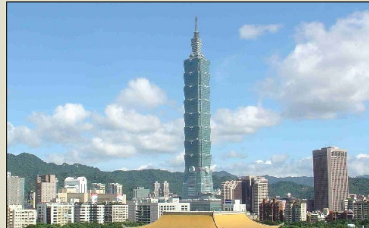
Taipei 101 (Taipei, Taiwan); C.Y. Lee and Partner, Architects, and Turner International Industries, Inc., project and construction management; concrete and steel megaframe, glass cladding; 2003-2004; height: 508 meters (1,667 feet), 101 floors; style: Neo-Regionalist Modern; building type: commercial office tower, skyscraper, shopping center.
