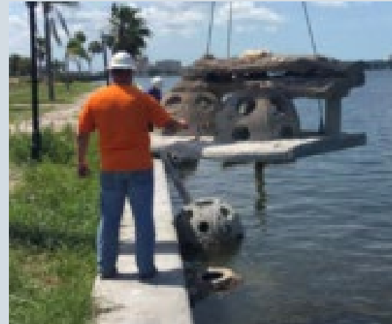
Reef Innovations Living Seawall units (Palmetto, 2016)
