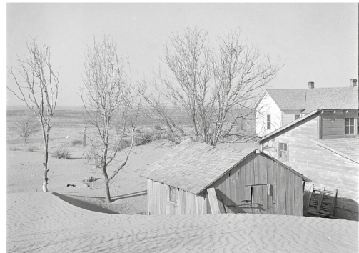
Photo credit Arthur Rothstein.
