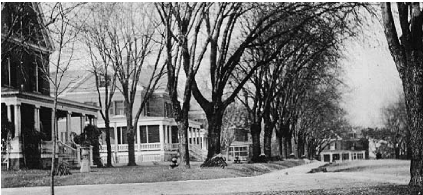
Officers' quarters along Grant Avenue, Fort Myer, Va., circa 1910-1915. Built between 1903 and 1909, the homes were sequentially numbered from right to left: Quarters One, Five, Six, and Seven.
