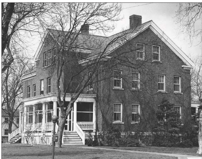
A view of Quarters Six while still configured as a duplex prior to the 1961 conversion. The renovation included major interior and exterior changes.
