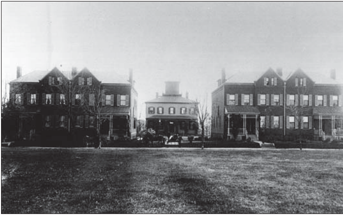
The old Signal Corps School “Observatory” centered between Quarters 11 and 12 at Fort Myer, Va. The observatory, constructed in 1876, contained twelve rooms for instruction and served as the post headquarters. The quarters were added during the 1890s.
