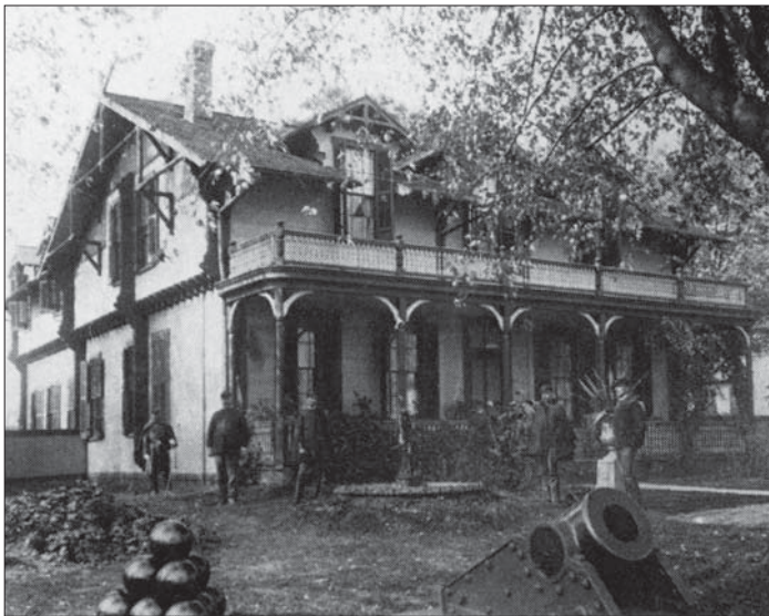
By 1892 the commanding officer's house had been slightly modified and was occupied by Lieutenant Colonel Guy V. Henry, left of center.
