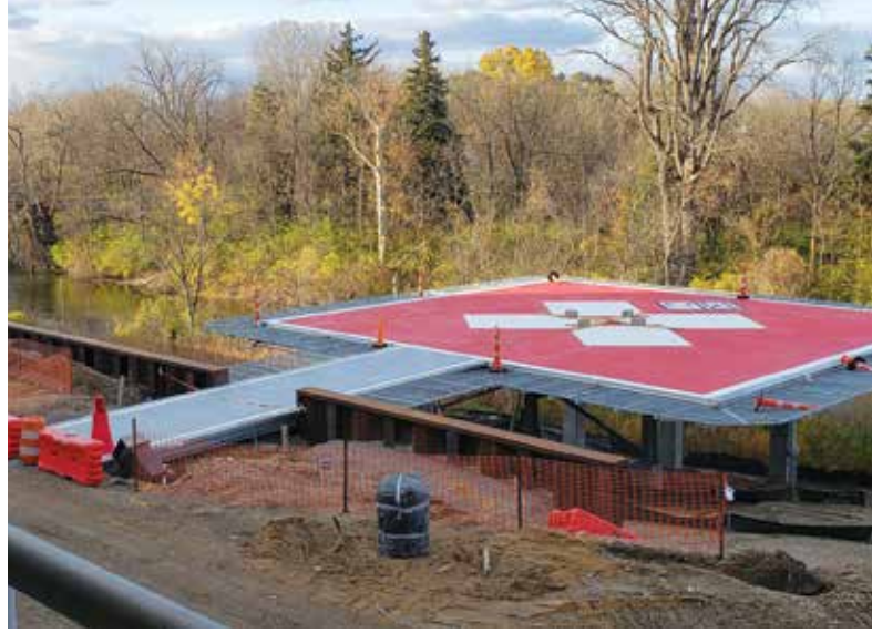
With hospital campus property a premium, the new helipad at McLaren Macomb has been constructed above the Clinton River.
