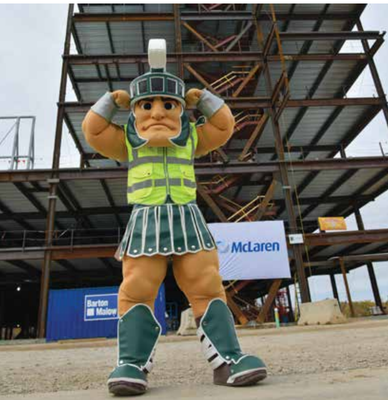
MSU mascot Sparty monitors progress of the new McLaren Greater Lansing hospital being constructed on the campus of Michigan State University in East Lansing.
