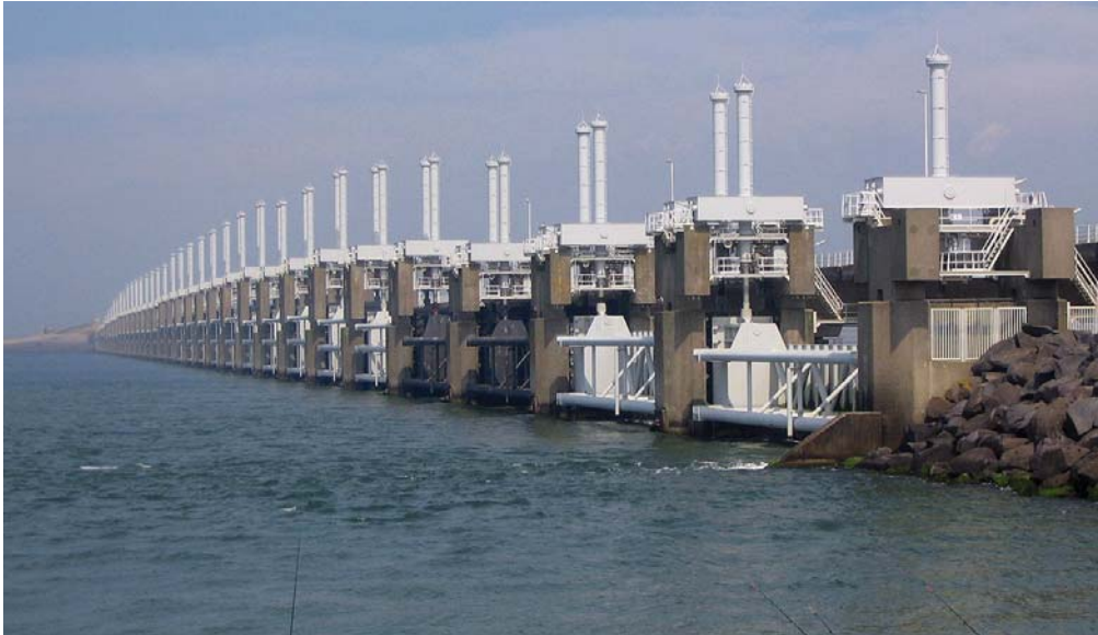
The disastrous North Sea Flood of 1953 spurred the government of the Netherlands to start work on the Deltaworks Project, a series of dams, dikes, sluices, locks, and levees to protect against another catastrophic storm surge. The Oosterschelde storm surge barrier (shown above) is the largest structure in the system, stretching nine kilometers and including sluice gates that are only closed during flood threats. A plaque on the structure reads: "Here the tide is ruled by the wind, the moon, and us (the Dutch)." PHOTO, VLADIMIR ŠIMAN
