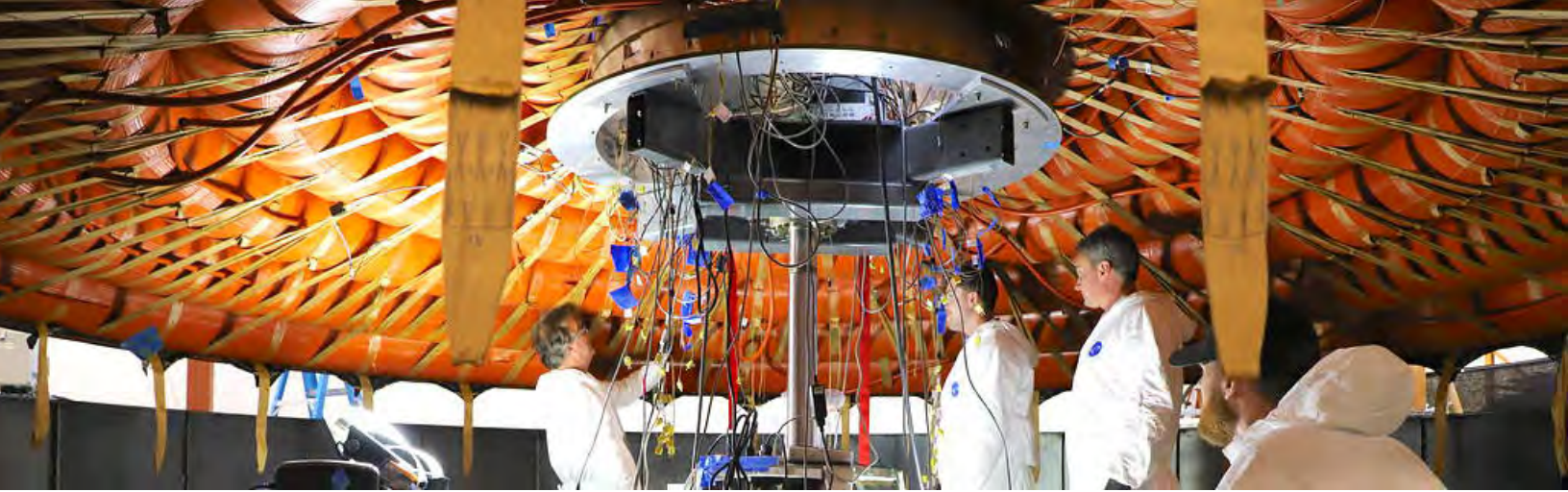
Engineers prepare for the flexible heat shield installation on the inflatable structure. The view is from bottom side, heat shield is on top. The gold straps hanging from the black triangles will be attached to the inflatable structure strapping and tensioned. Credit: NASA's Langley Research Center.
