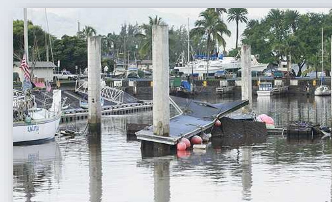
Images show damage in the Hale'iwa Harbor on O'ahu from the 2011 Tohoku, Japan tsunami. 2 m runup height. Image credit: Mader Consulting Co.
