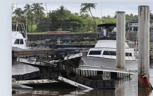
Images show damage in the Hale'iwa Harbor on O'ahu from the 2011 Tohoku, Japan tsunami. 2 m runup height. Image credit: Mader Consulting Co.
