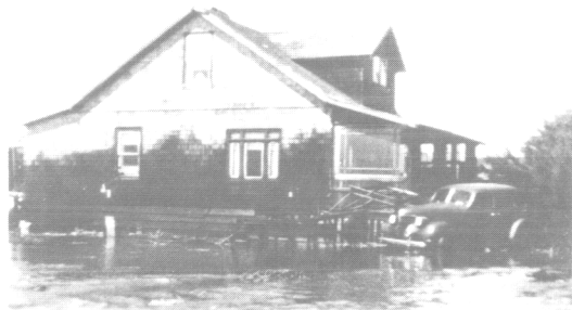
Figure 13. Home at Half Moon Bay showing water height to its windows from the April 1 tsunami. Photo taken about 10:30 A.M. by Howard Anderson (Magoon, private collection).
