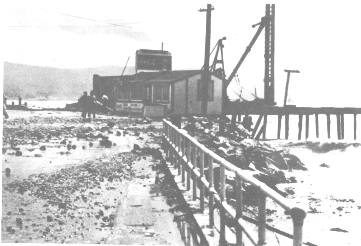
Figure 15. Rocks carried on to the road at Half Moon Bay pier. Picture taken by Manuel Sousa at about 11 A.M. Note continuing wave action. (Magoon, private collection.)
