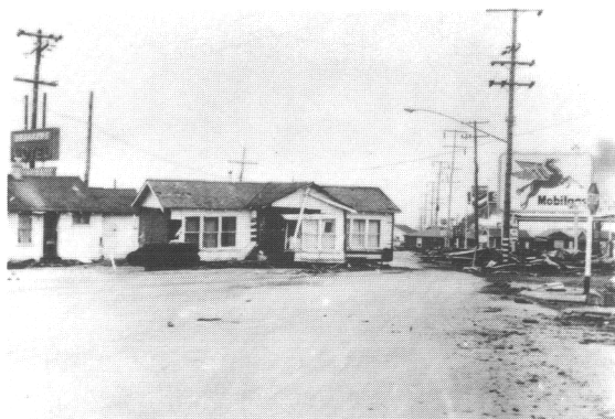
Figure 27. Office and motel unit from Van's Motel block Highway 101. These structures floated from their foundations and damaged units in the next door Breaker's Motel. (Photo credit: U.S. Army)
