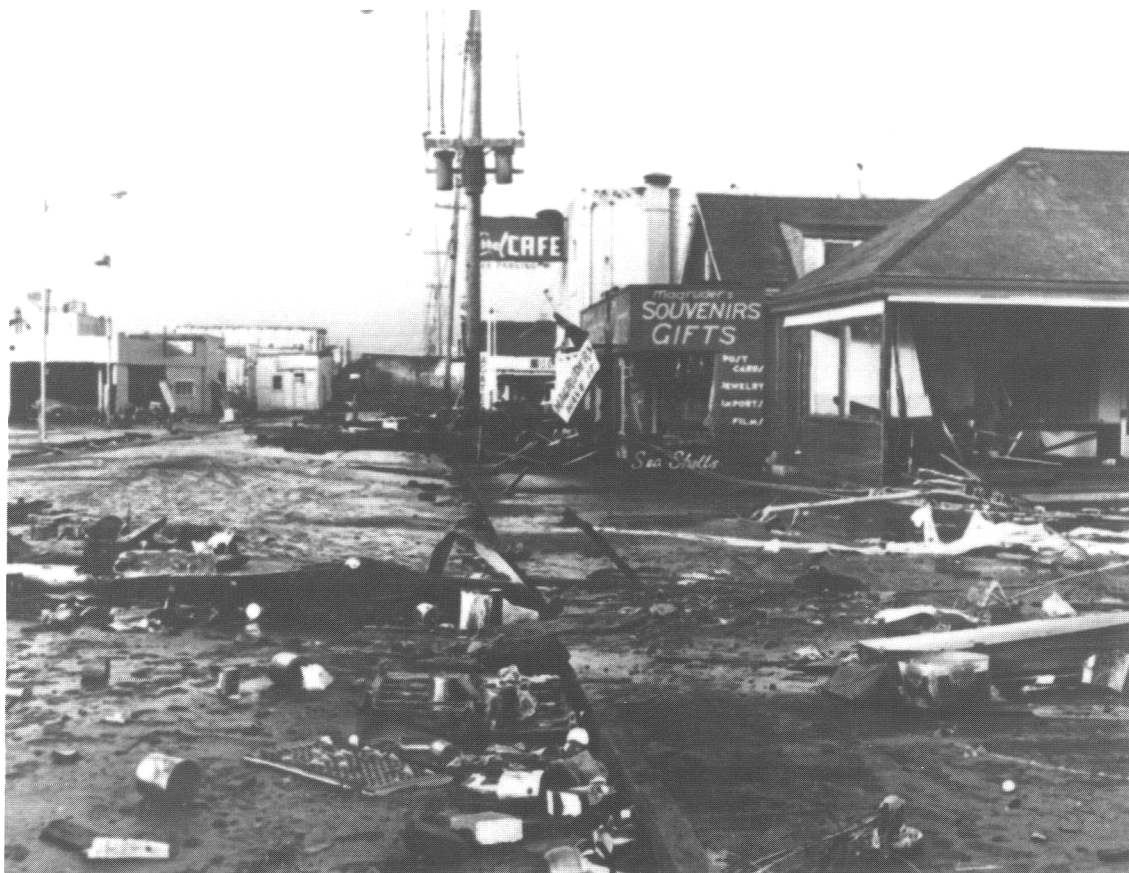
Figure 29. Second Street looking west from L Street. Note typical debris in the foreground and buildings moved into the street in the background. (Used by permission, Wallace Griffin, Crescent City Printing Co.)
