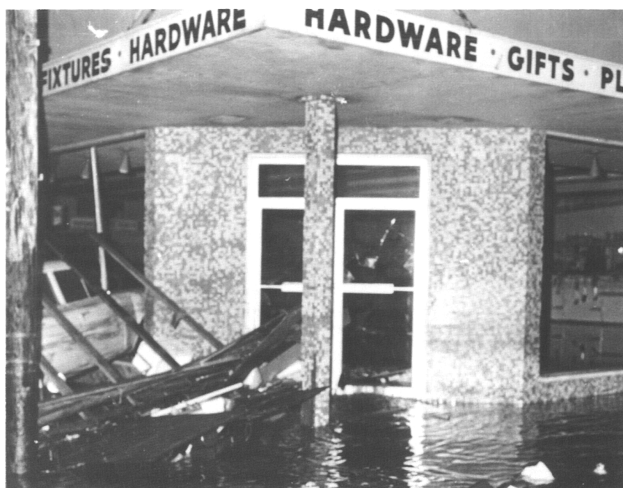
Figure 25. Nielsen's Hardware at 3rd and I Street, Crescent City, where water was four to six feet high. (Used by permission, Wallace Griffin, Crescent City Printing Co.) Note car intruding through the window. Damage is increased by floating projectiles such as automobiles, logs, and boats.
