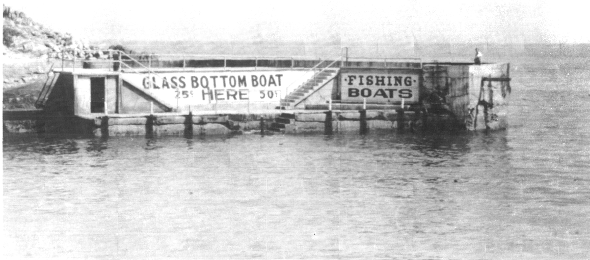
Figure 16. Municipal swimming pool at Pacific Grove, California, where high water from the April 1, 1946 tsunami reached the bottom of the word BOATS and flooded the dressing room three feet deep. A man fled up the steps ahead of the single surge. (Magoon, private collection.)
