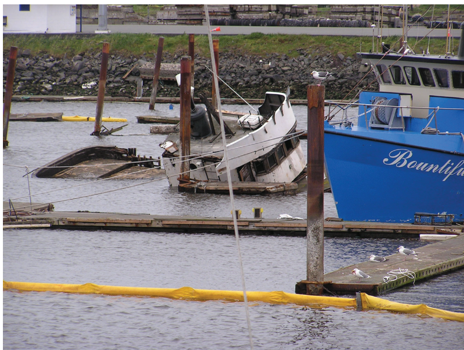
The 2011 Honshu, Japan, tsunami caused extensive damage in a number of harbors in California, including $20 million in damage at Crescent City. Photo credit: Rick Wilson, California Geological Survey.
