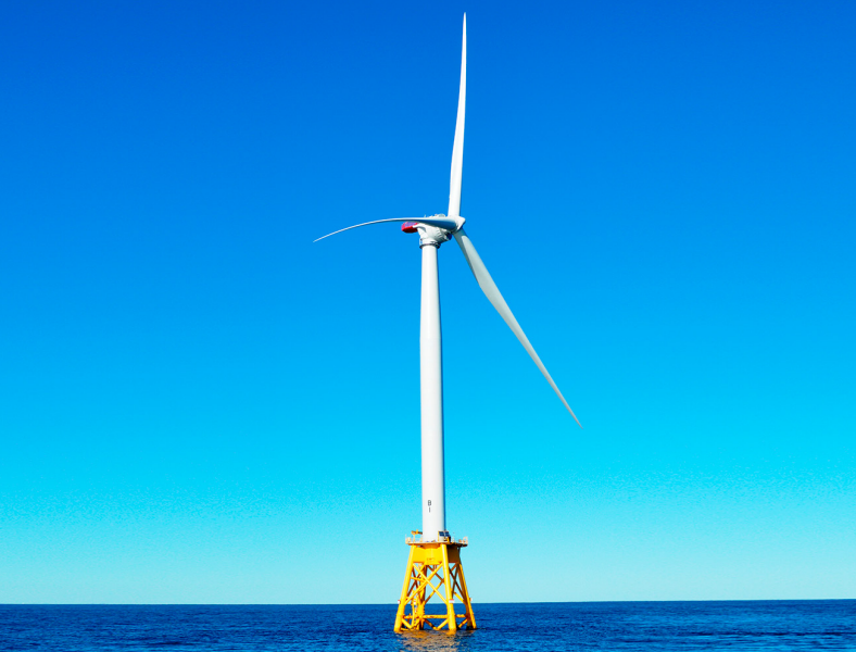
Block Island Wind Farm, 3 miles off the coast of Rhode Island.
