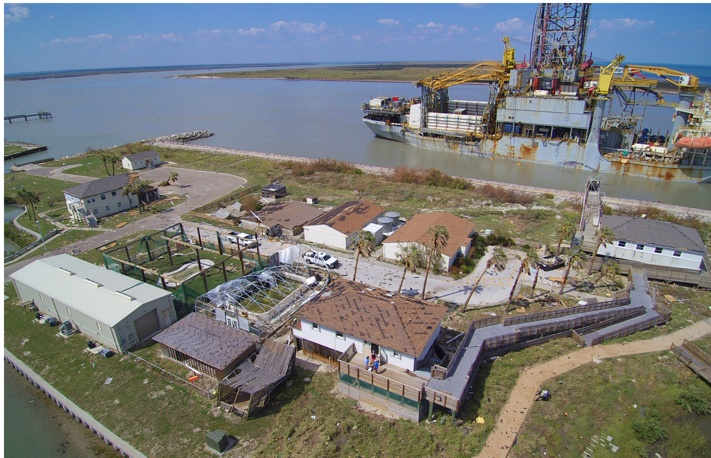
Damage to facilities at the Mission-Aransas National Estuarine Research Reserve in Texas following Hurricane Harvey.
