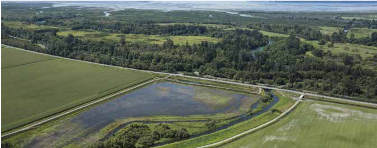
NOAA's efforts to restore marshland and set back dikes on the Skagit River, WA are helping to protect neighboring farmland and roads from flooding while also improving fish access to new and existing habitat. Photo Credit: Marlin Greene/One Earth Images
