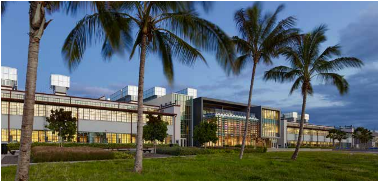
The Inouye Regional Center (IRC) is located on historic Ford Island, Naval Station Pearl Harbor, Honolulu, Hawaii. The IRC combines new facilities with the historic preservation of four historic buildings culminating into a campus which is environmentally sustainable, state of the art and Leadership in Environmental and Energy Design (LEED) Gold Certified.
