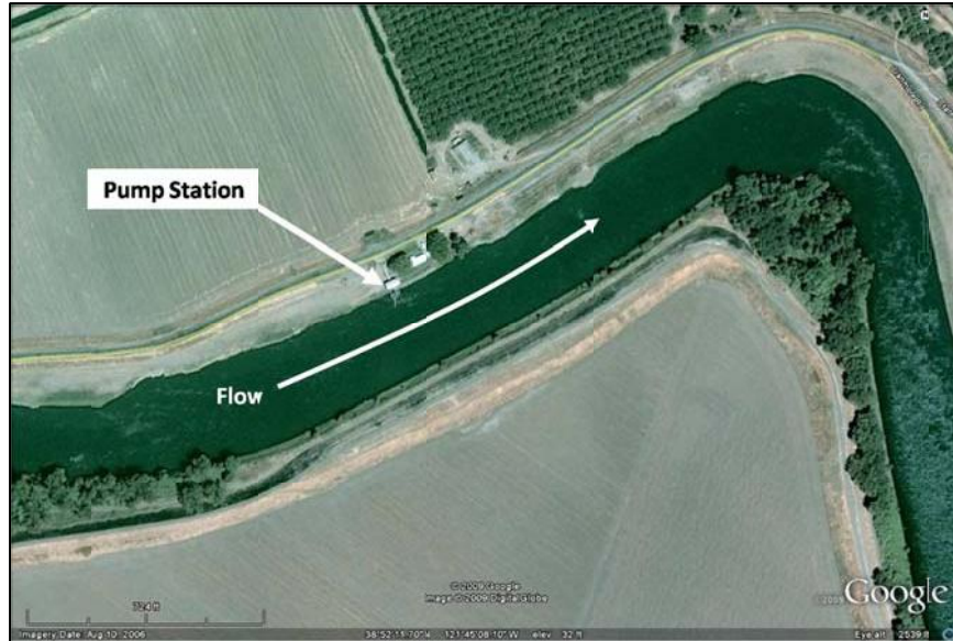
Figure 36. Location of the State Ranch pump station on the Sacramento River.
