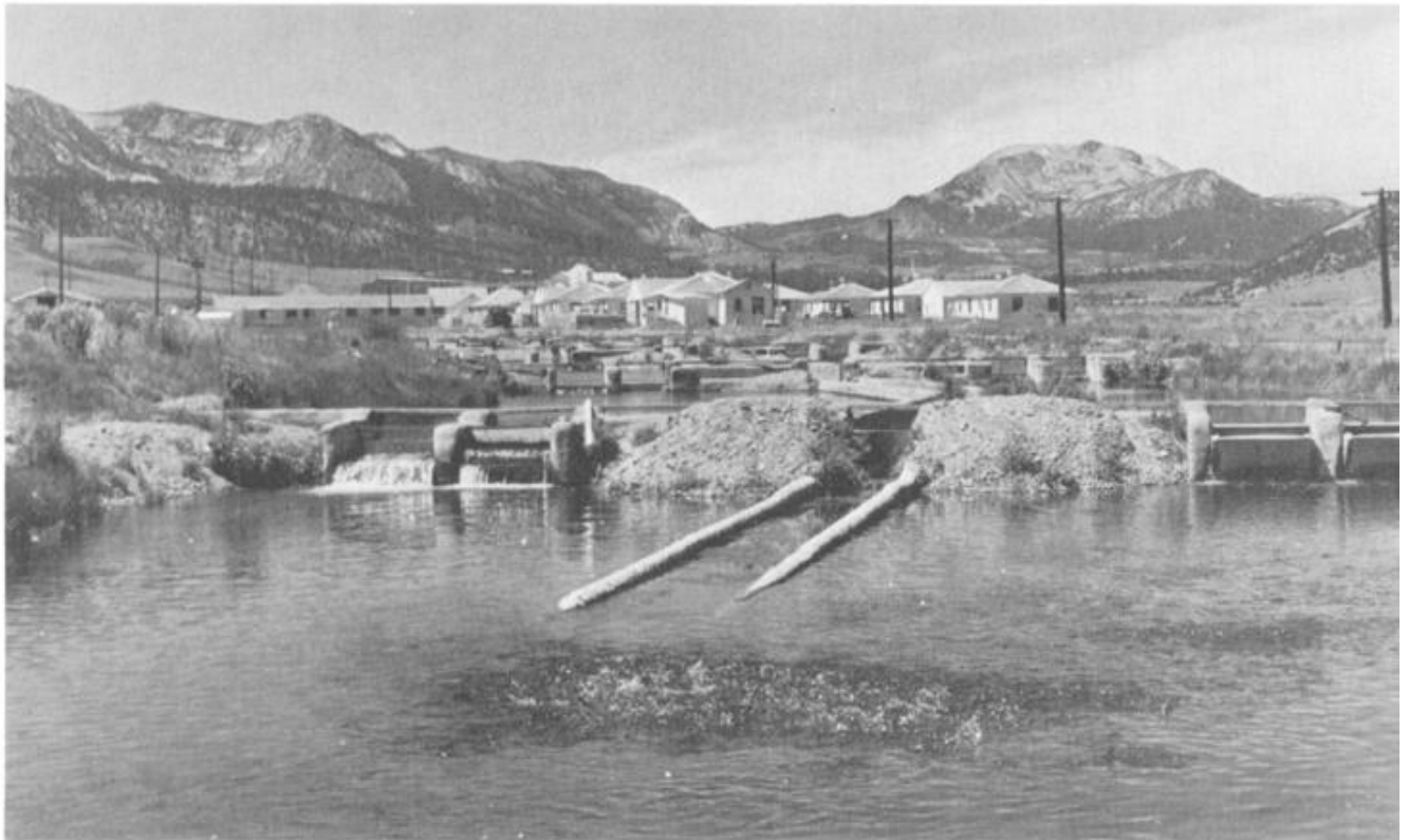
FIGURE 36. Hot Creek Hatchery, 1959.
