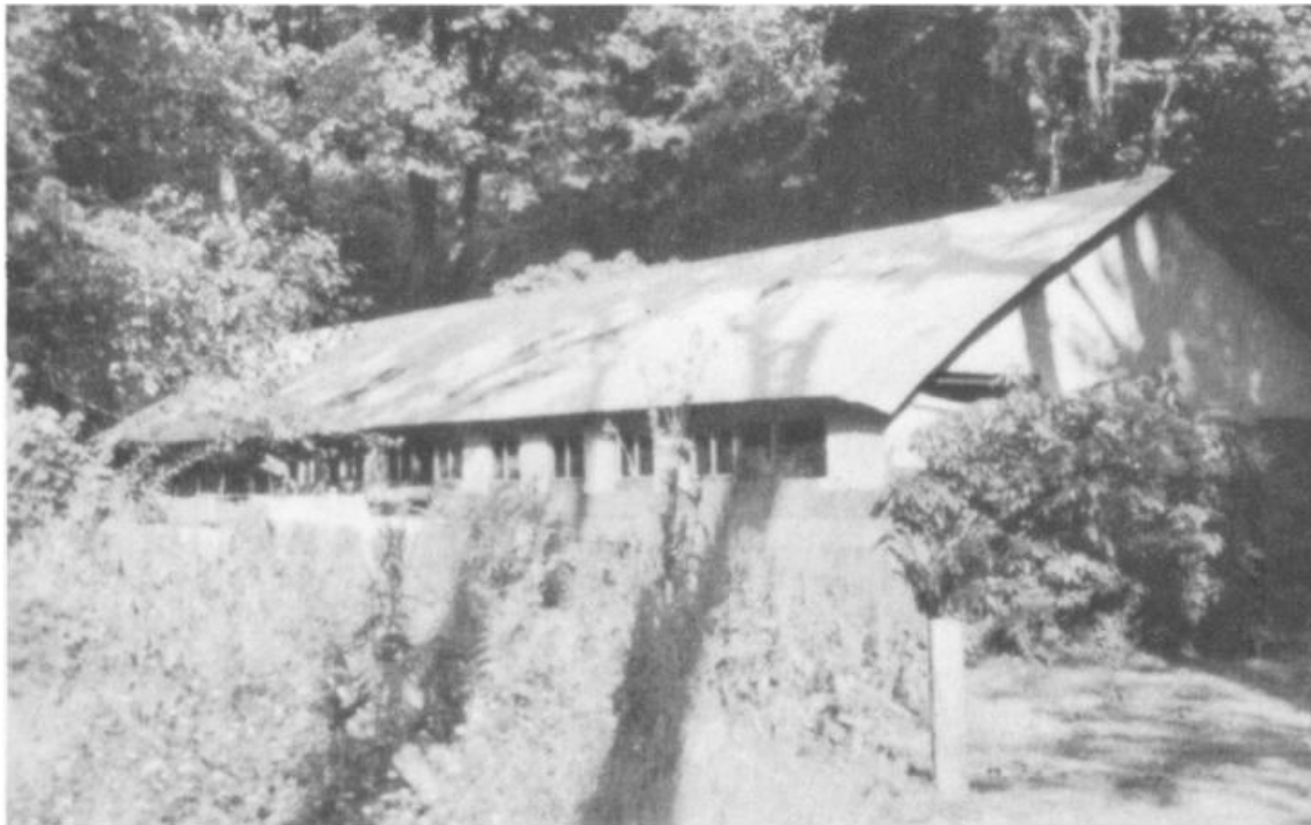
FIGURE 37. Old hatchery building, Prairie Creek Hatchery.
