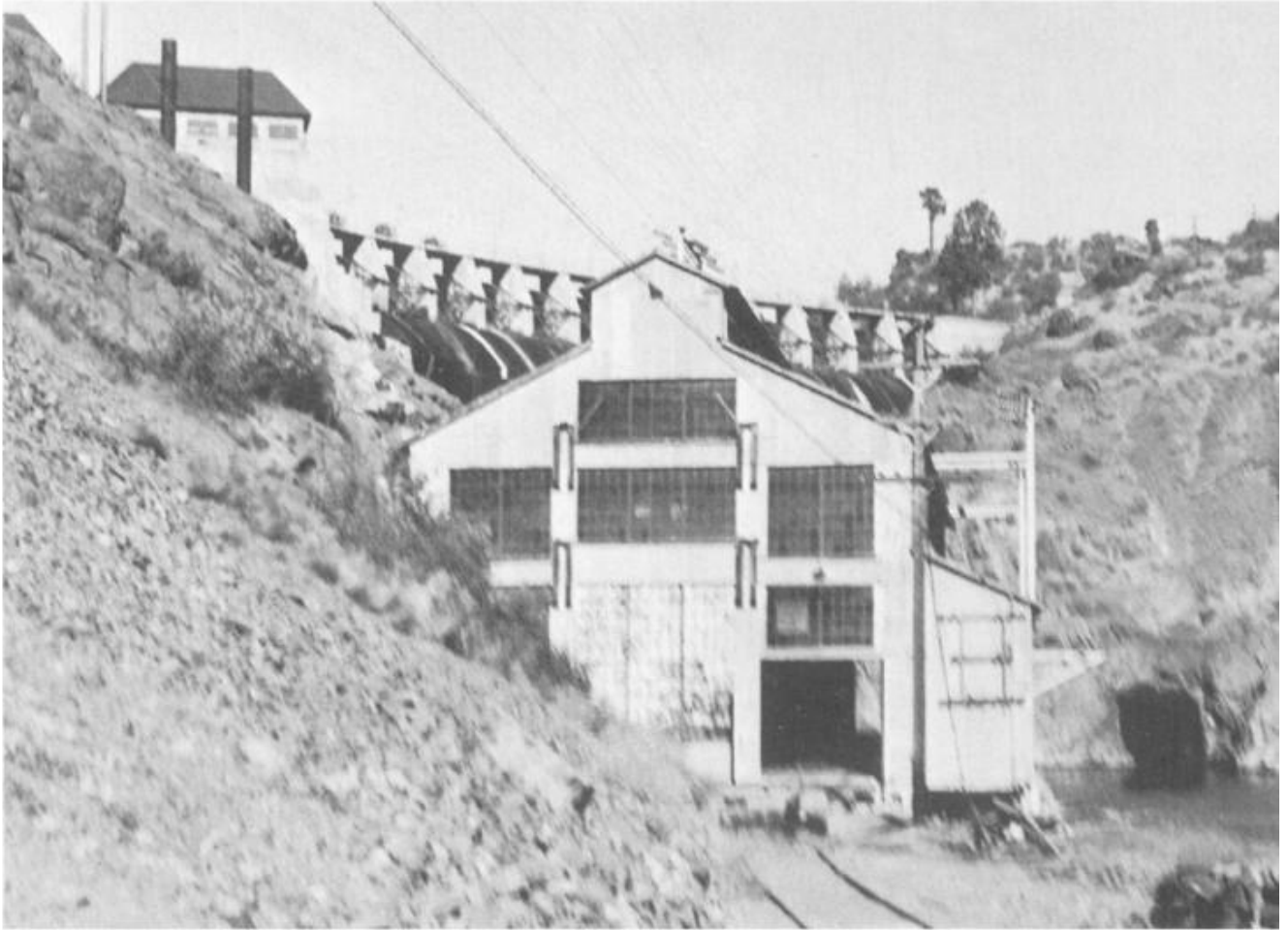
FIGURE 13. Copco Dam and Powerhouse.
