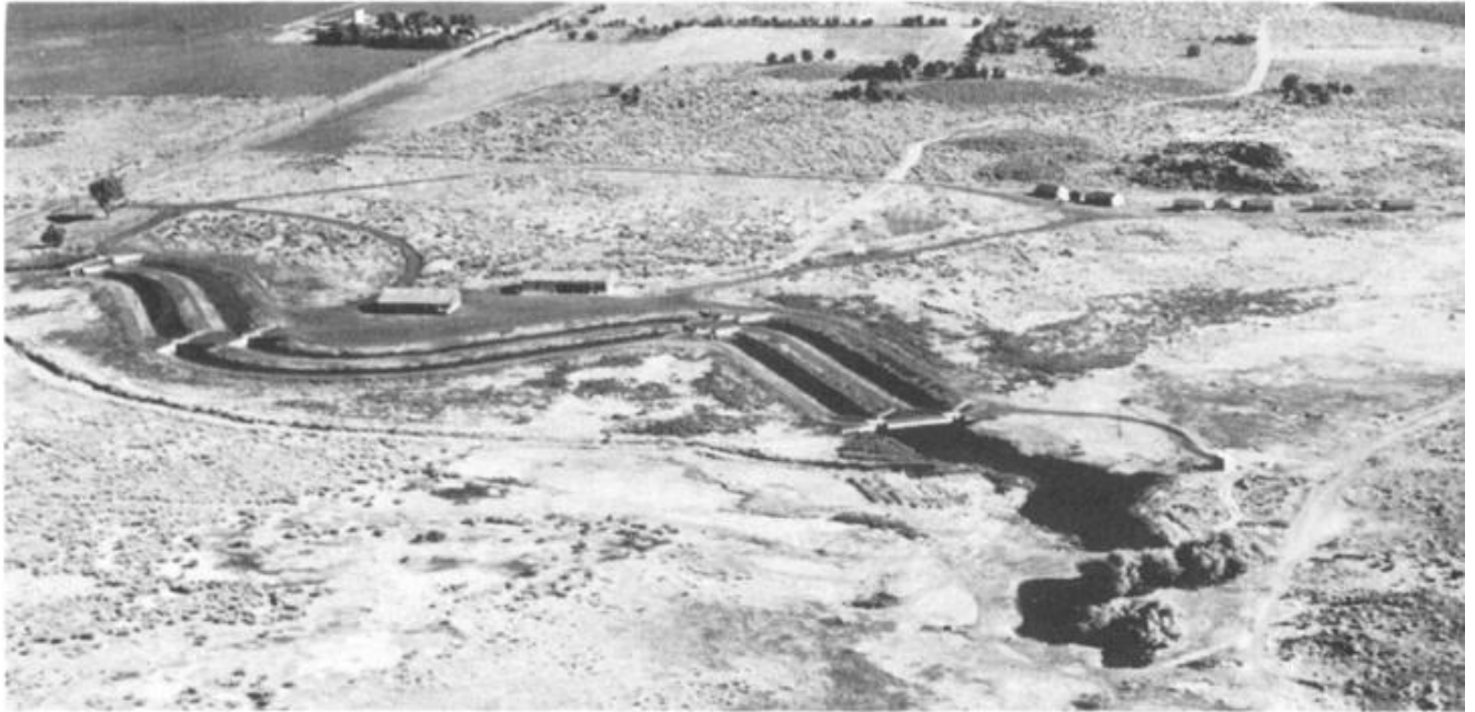
FIGURE 51. Aerial view of Fish Springs Hatchery shortly after completion in 1952, showing spring area with six earthfill ponds in foreground, food storage and utility buildings in center, and employees' houses on right.
