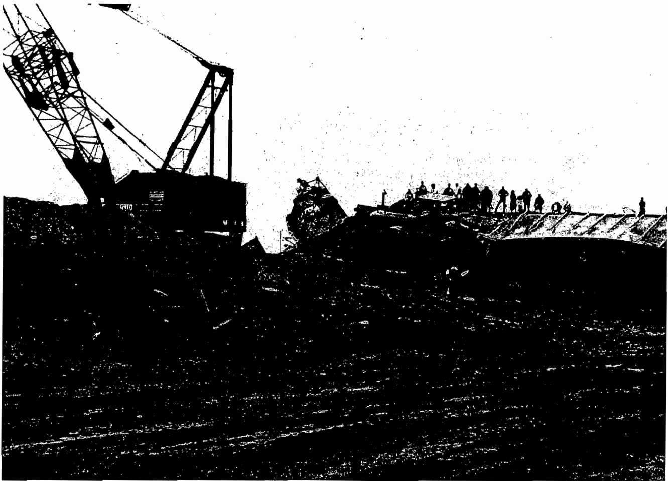
Figure 9.--Equipment used to move cars to west side of track.
