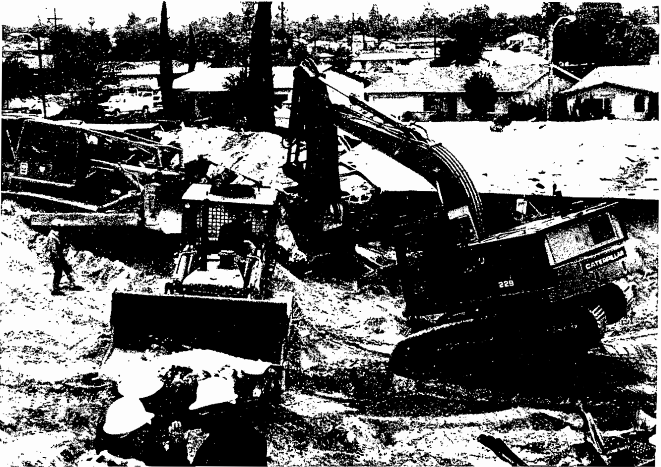
Figure 7.--Equipment used during wreckage removal.
