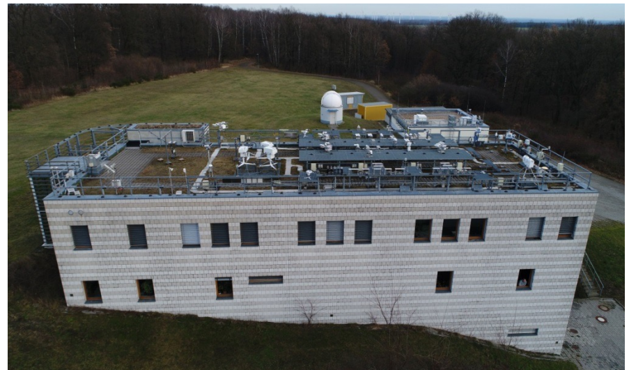
DWD – BSRN station and Regional Radiation Center WMO at Meteorological Observatory Lindenberg
