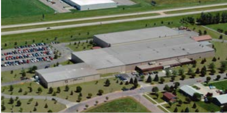
Brookings, SD Manufacturing Facility
