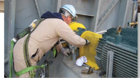
Coupling & Sheave Alignment
