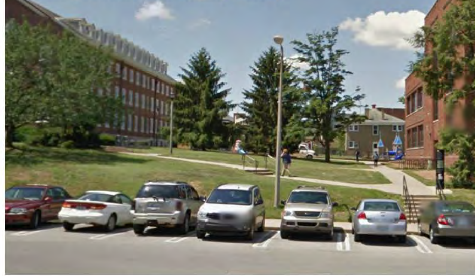
SITE 16 : BRECKINGRIDGE HALL AND FUNKHOUSER LAWN (looking south from Library Drive)
