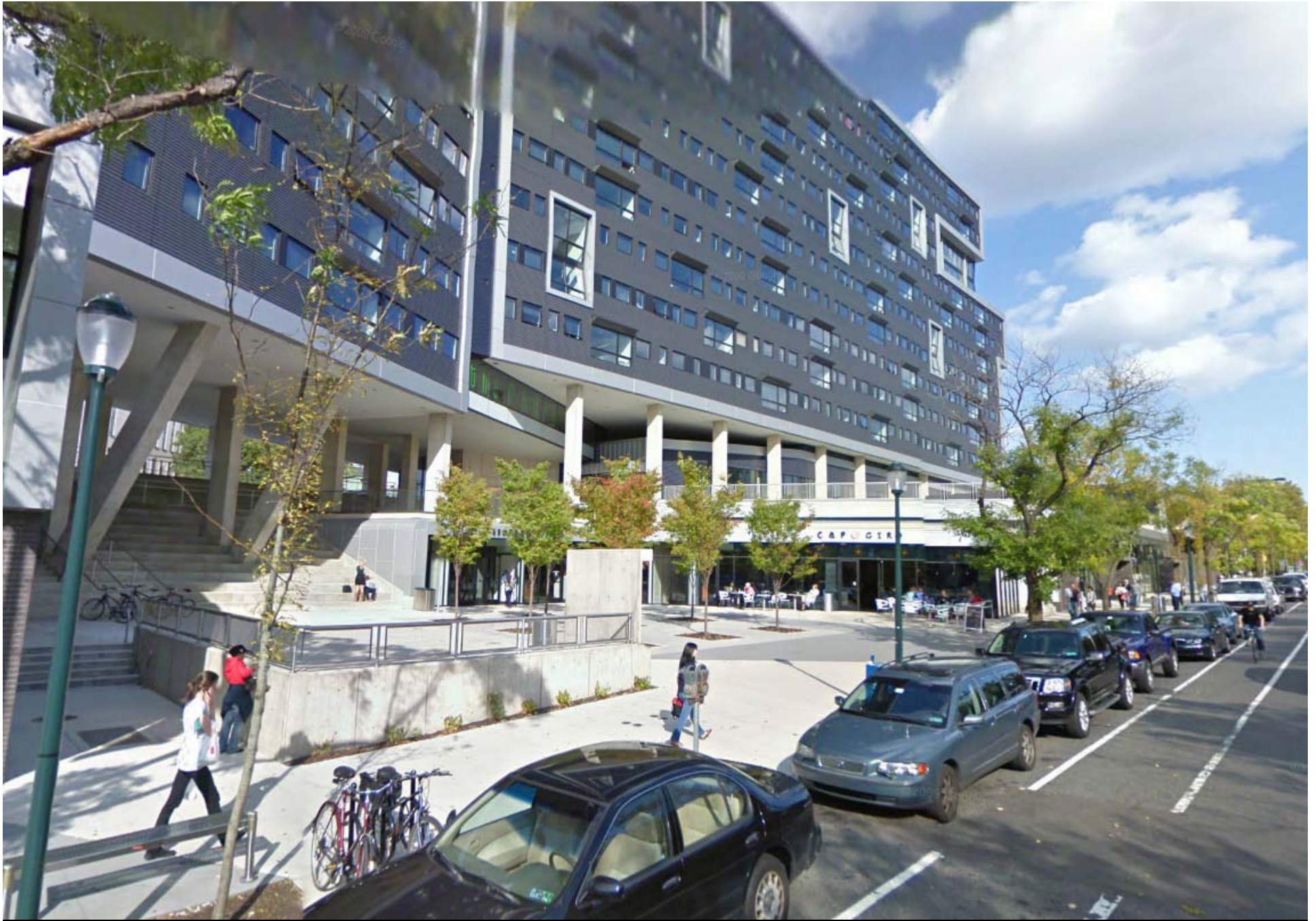
Radian - Street View West
