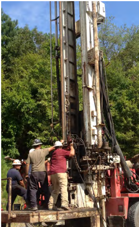
Installing tubing and packer in the Crossrock No. SS-#1 test well.
