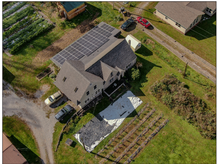
Photo by Jones Aerial Photography Southdown Farm in Letcher County added solar in 2019, working with Mountain Association to receive nearly $20,000 in grant funding. The system allows them to save approximately $2,600 per year.
