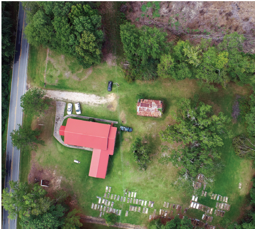
Researchers at Penn's Center for the Preservation of Civil Rights Sites and Tuskegee University are collaborating on stabilizing the structure and developing an interpretation plan for the historic Armstrong School.
