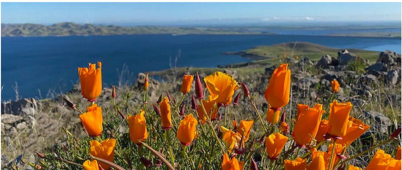
In summer of 2022, Reclamation broke ground on this $1B project, the largest Safety of Dams project to date, at B.F. Sisk Dam located on the west side of California’s Central Valley. Reclamation’s Safety of Dams Program started in 1978 to ensure its dams do not present unreasonable risk to people, property, and the environment.
