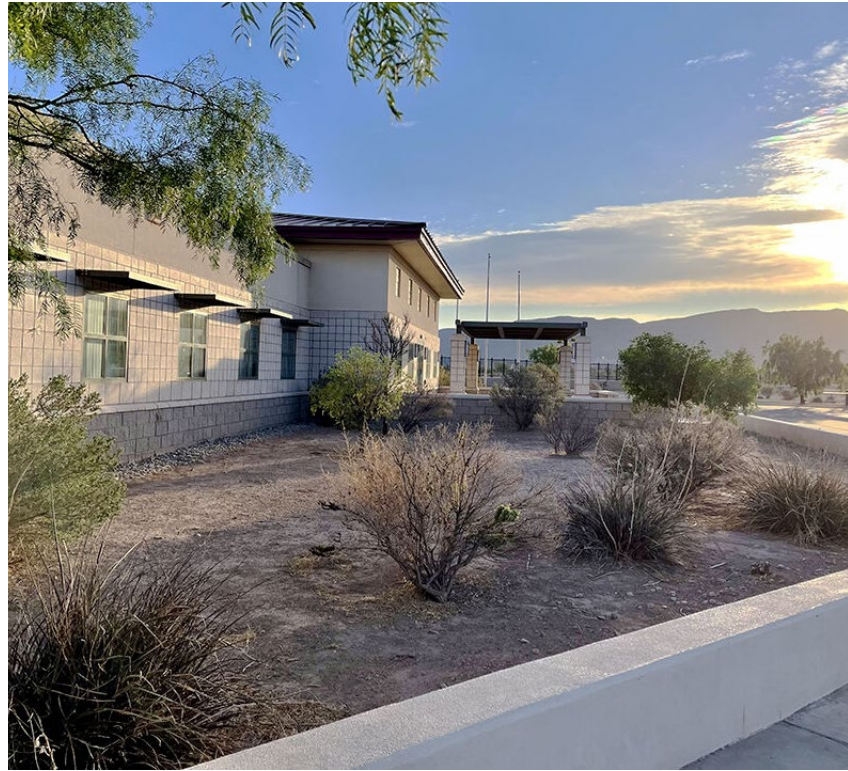
Reclamation's Brackish Groundwater National Desalination Research Facility in Alamogordo, New Mexico.
