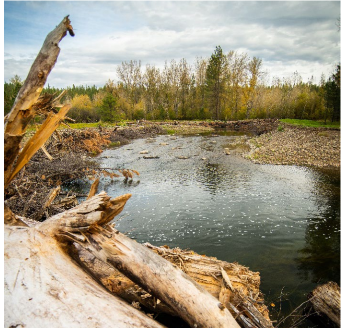
The Bird Track Springs reach of the Grand Ronde River in Oregon has been heavily degraded by multiple historical practices resulting in poor aquatic and floodplain habitat. Reclamation, along with Federal and Tribal partners, is implementing a habitat enhancement project in the area. One activity is the placement of large logs, as seen in this image, to help retain banks and provide habitat for fish.
