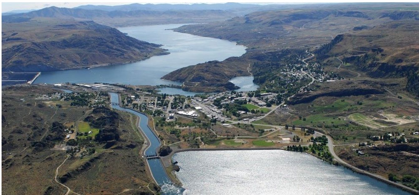
Twelve of the world's largest pumps lift water over 280 feet up from the reservoir (Franklin D. Roosevelt Lake) created by Grand Coulee Dam in Washington into a feeder canal and Banks Lake (pictured here). This water is then delivered to over 10,000 farms.
