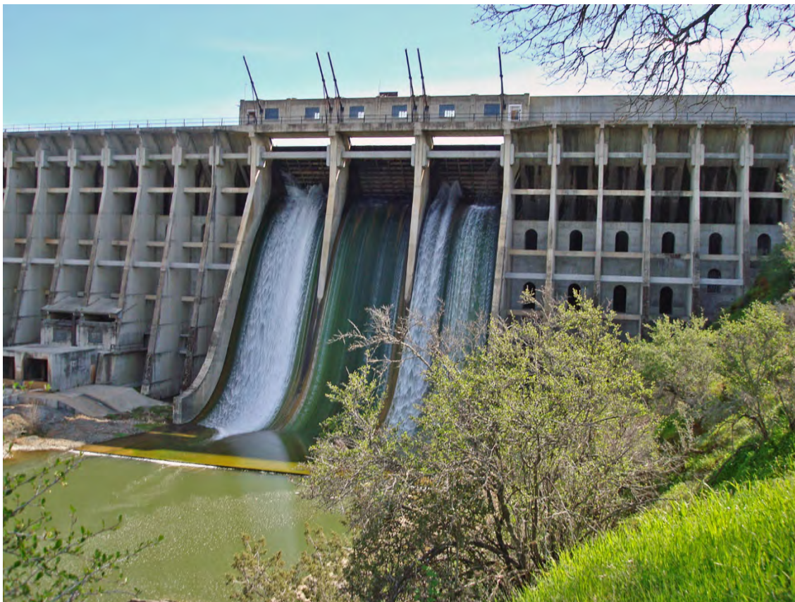
Stony Gorge Dam, Northern California Area Office, Mid-Pacific Region.
