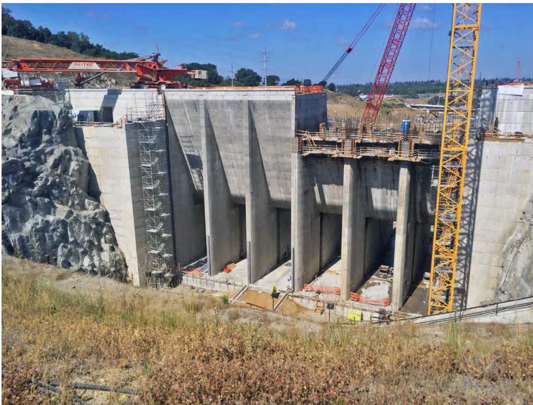
Folsom Dam Auxiliary Spillway Control Structure, Central Valley Project, Mid-Pacific Region.
