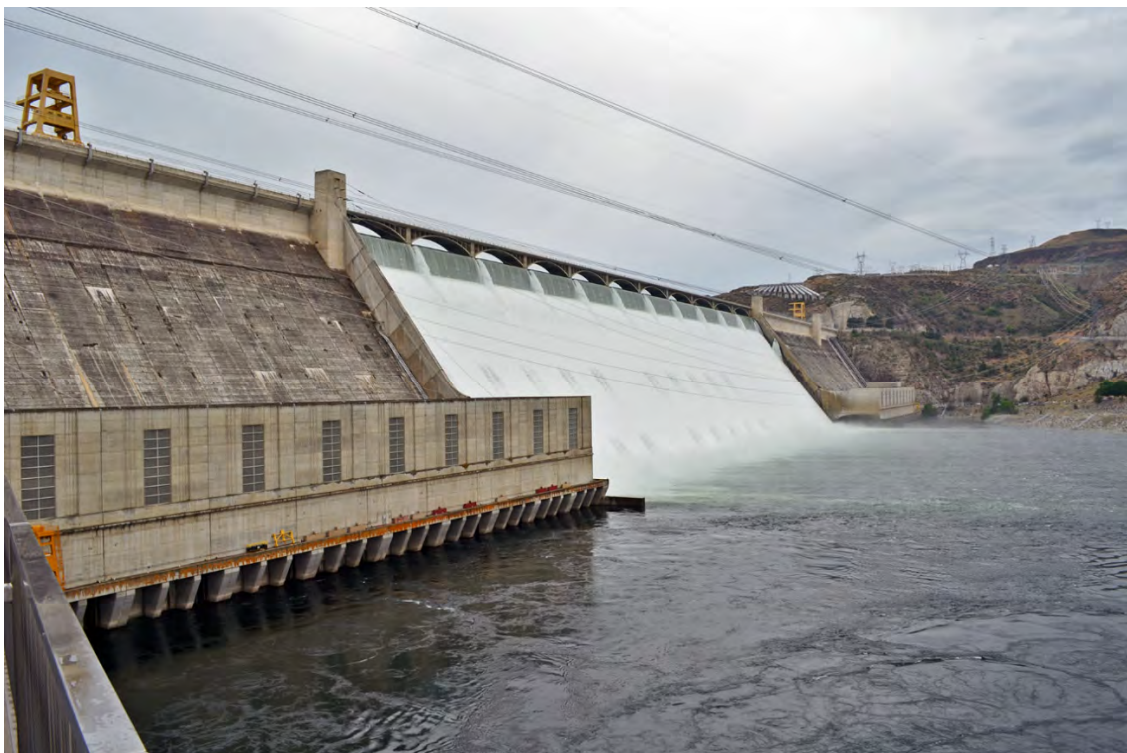
Grand Coulee Dam, Columbia Basin Project, Pacific Northwest Region.
