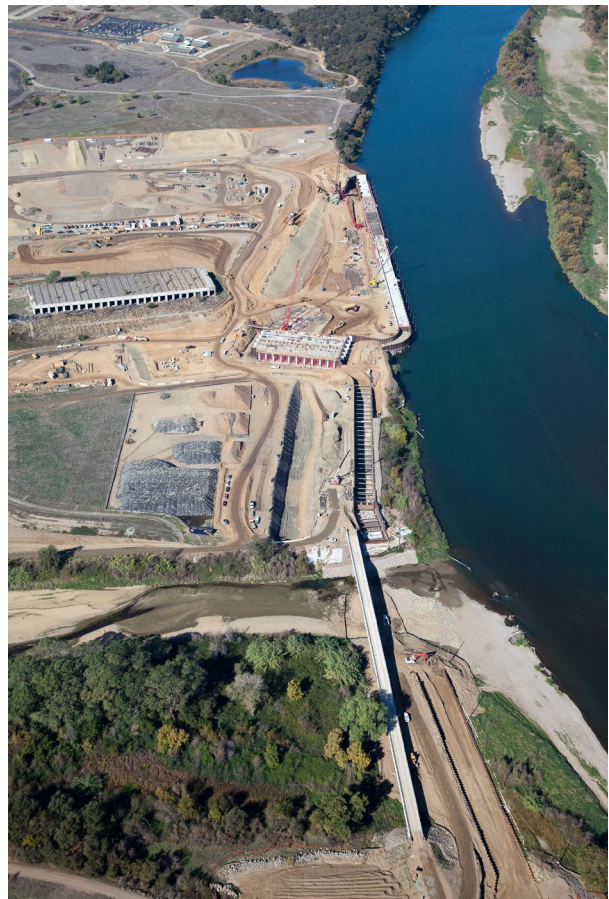
The extensive size of the project shows in this aerial view.
