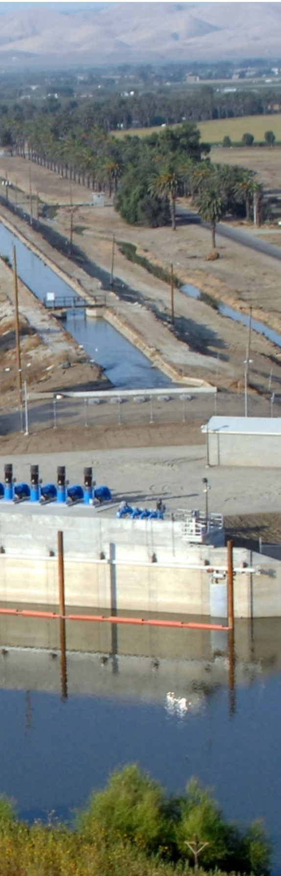
Pumps draw water through the new fish screen into an irrigation canal.
