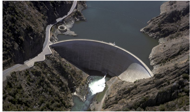
Monticello Dam, with Glory Hole Spillway
