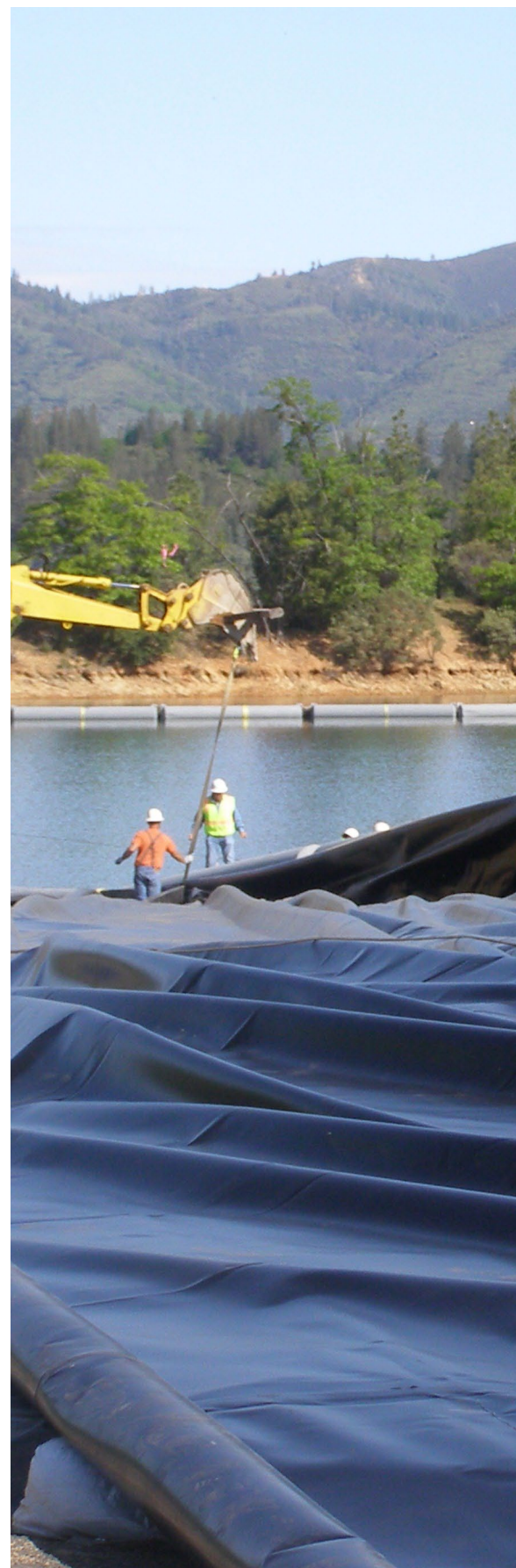
Workers install a replacement temperature control curtain in V
