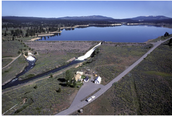
Boca Dam and Reservoir
