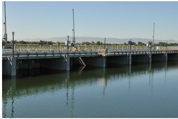
Water passes through the new fish screen.
