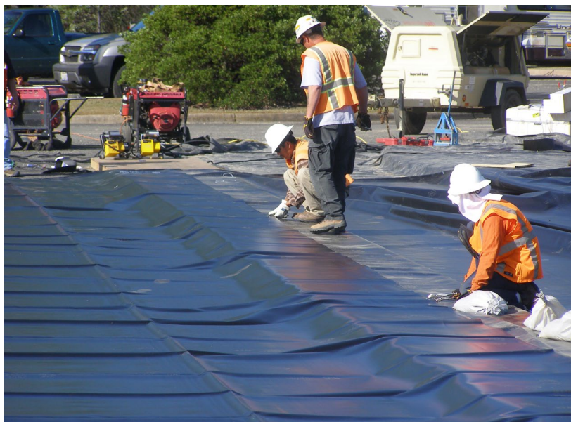
Workers prepare temperature control curtain for deployment.
