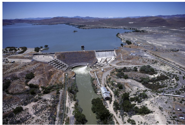
Lahontan Dam and Reservoir
