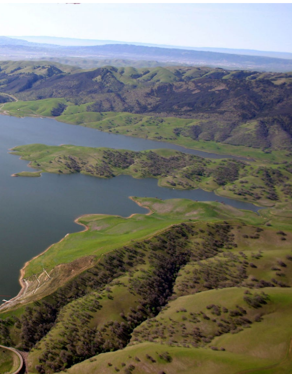
Center photos: Top : Shows construction work on Los Vaqueros Reservoir; Bottom : An aerial view of the entire reservoir.
