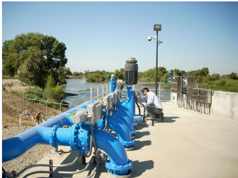
Pumps draw water through the new fish screen into an irrigation canal.
