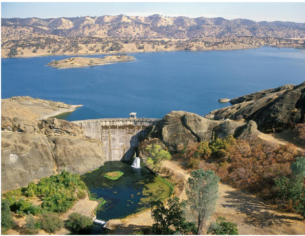
East Park Dam
