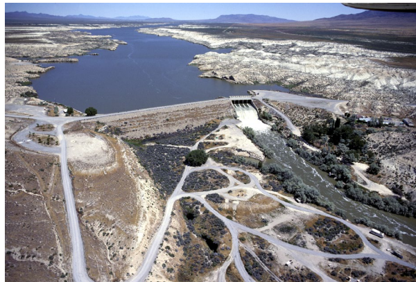
Rye Patch Dam and Reservoir
