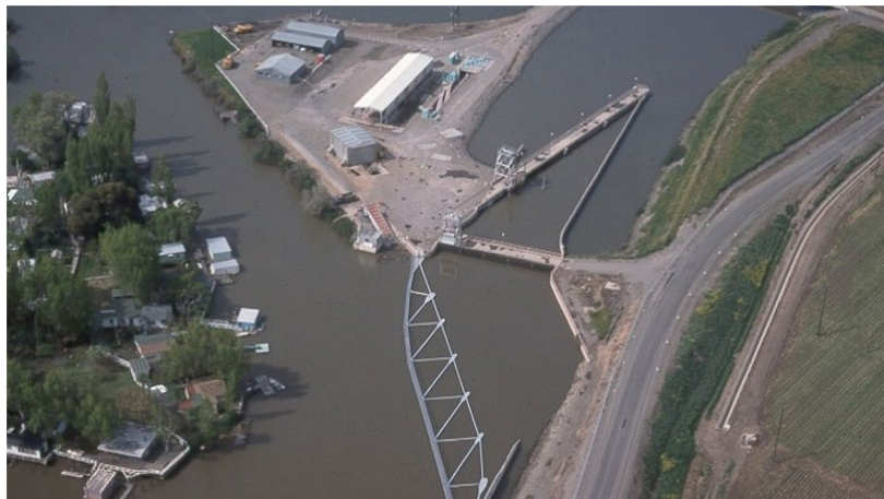
The Tracy Fish Collection Facility protects fish natural to the Sacramento-San Joaquin Delta from the nearby C.W. "Bill" Jones Pumping Plant.
