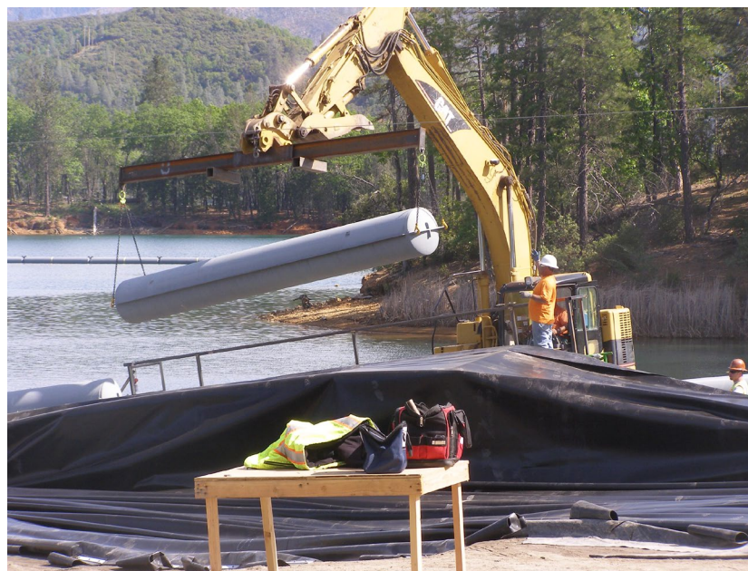
A crane is used to lift a piece of the temperature control curtain.
