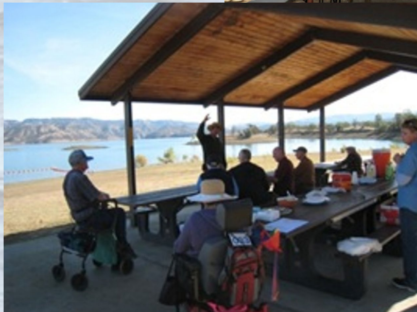
A completed accessibility project at Lake Berryessa.
