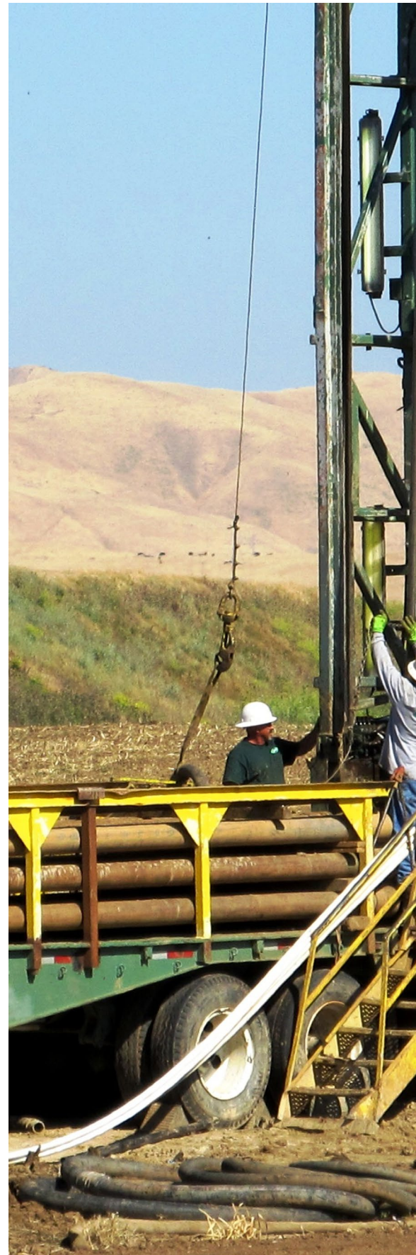
Workers drill a well near Los Banos, California.
