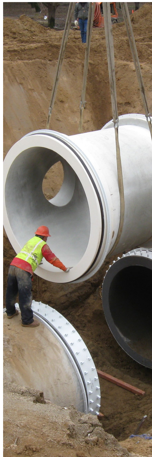
Workers lower pipe that is part of an interconnection between
