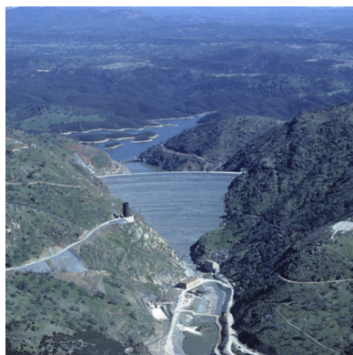
New Melones Dam and Reservoir
