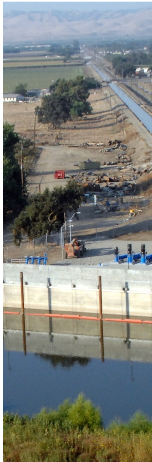
The completed Patterson Fish Screen Project.
