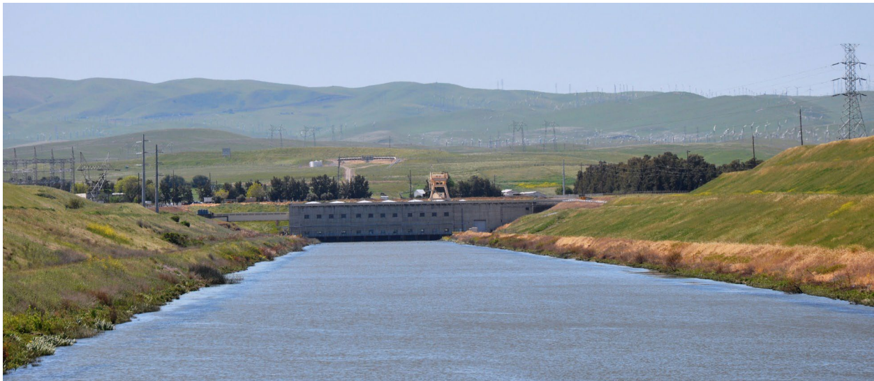
The C.W. "Bill" Jones Pumping Plant is located at the southern end of the Sacramento-San Joaquin Delta.
