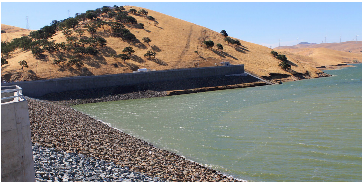
The Los Vaqueros Dam was raised by 34 feet to a height of 521 feet.
