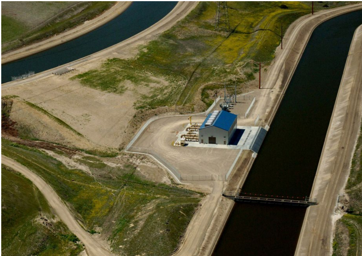
The photo above and the diagram below show the Intertie and how the facility functions. On the left side of both the photo and diagram is the California Aqueduct and on the right side is the federal Delta-Mendota Canal. The building next to the DMC is a pumping plant. Water can flow downhill through underground pipes (shown in the diagram) from the higher California Aqueduct to the DMC. The pumping plant also can transfer water from the DMC, uphill, to the California Aqueduct.
