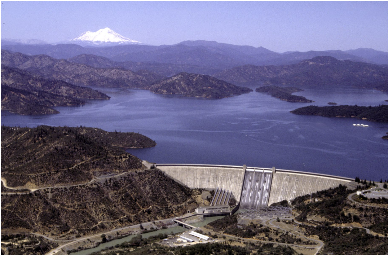
Shasta Dam in Northern California is the subject of studies analyzing whether the structure should be raised.
