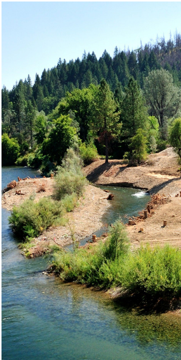
Trinity River Restoration work includes channel rehabilitation.
