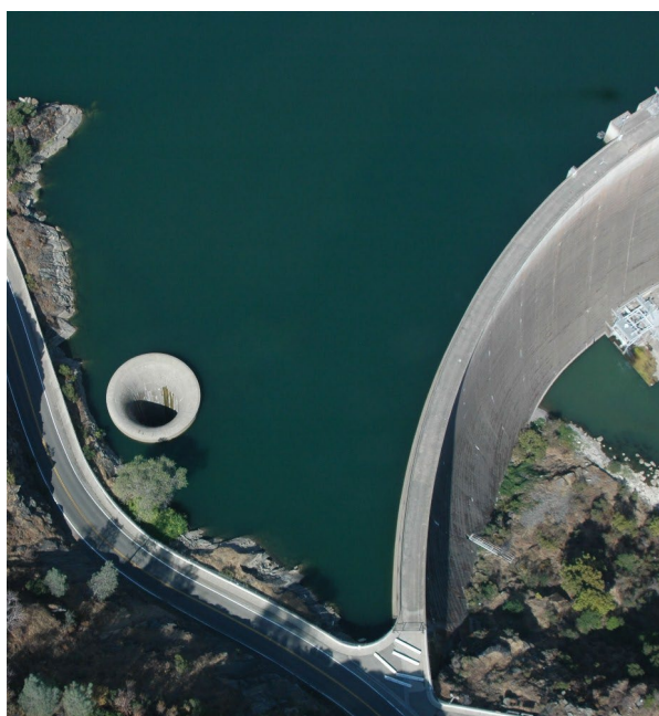
Monticello Dam, with a morning glory spillway, in the Solano Project.
