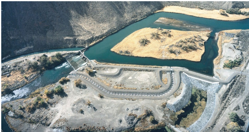
Derby Dam in the Newlands Project.
