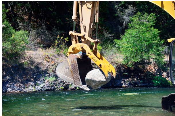
Above and below: Changes in the Trinity River to improve fish habitat include creating an island and placement of boulders.
