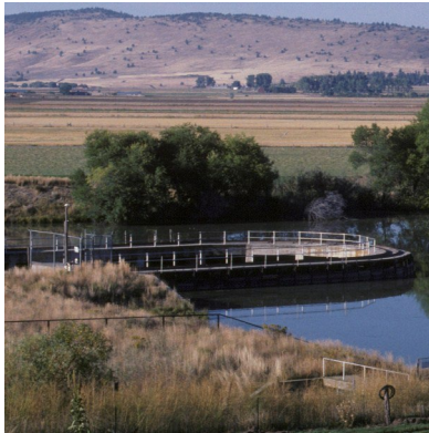
Lost River Diversion Dam in the Klamath Project.
