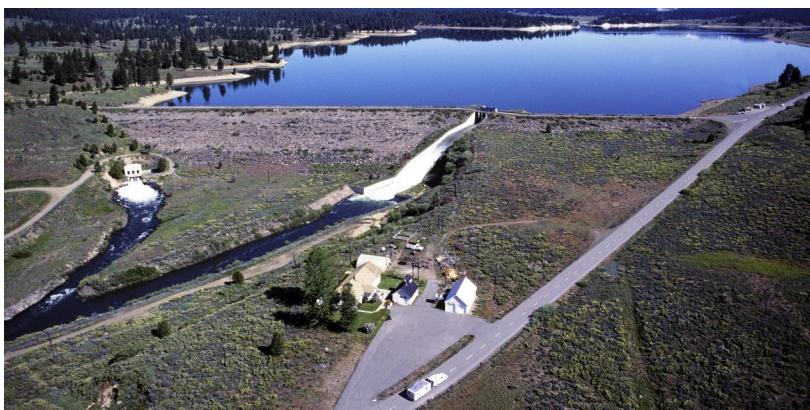
Boca Dam in the Truckee Storage Project.
