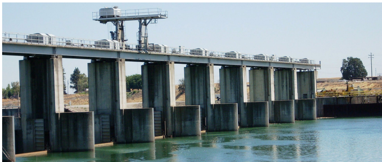
Red Bluff Diversion Dam with closed gates.
