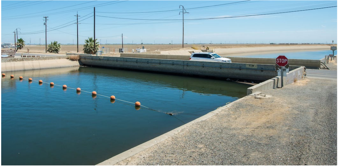
Photo of Delta-Mendota Canal showing subsidence. Located along the west side of the San Joaquin Valley, the Delta-Mendota Canal is essential for irrigation supply as part of the San Luis Unit and CVP's Delta Division. Courtesy of California Department of Water Resources.
