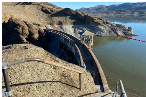
When the reservoir was at its lowest since 1977 due to ongoing drought conditions last August, the area was closed to allow for inspections at East Park Dam in Colusa County.
