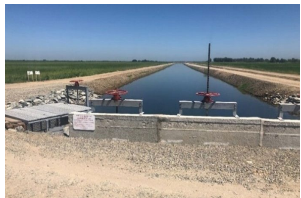
Lower Schwind Canal and Head Gate.
