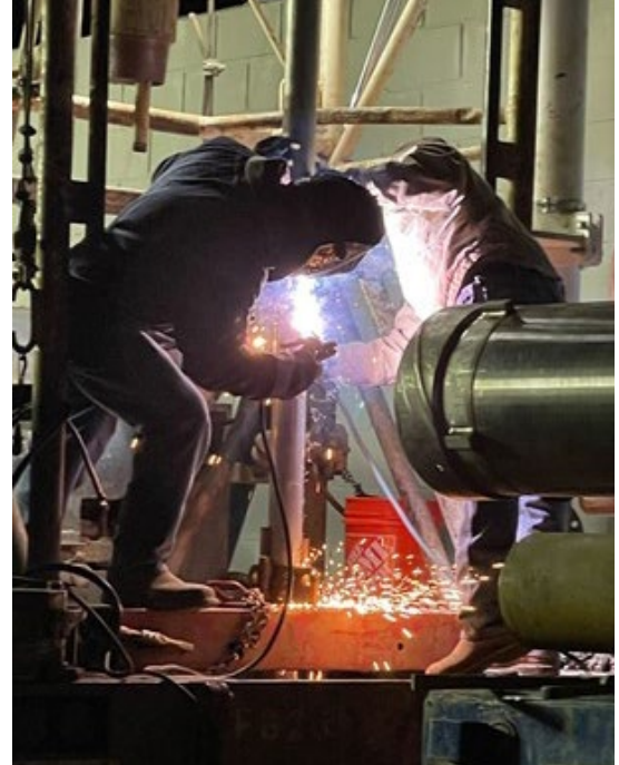
Welders working on the infrastructure for the new wastewater purification facility
