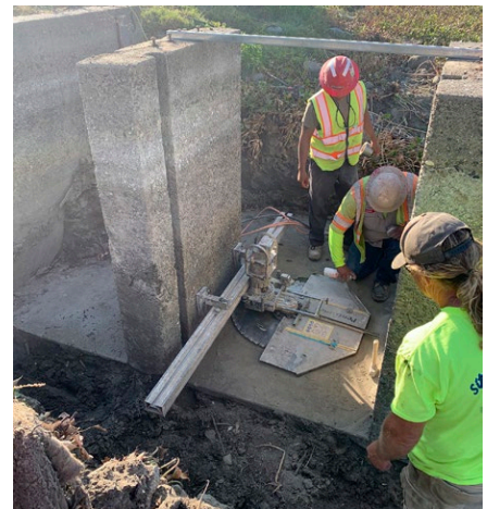
SJRRP improved fish passage by removing a weir in the San Luis National Wildlife Refuge in Merced County.
