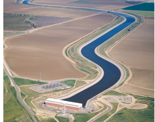
An aerial view of the California Aqueduct San Luis Canal in Merced County with Dos Amigos Pumping Plant in the foreground.
