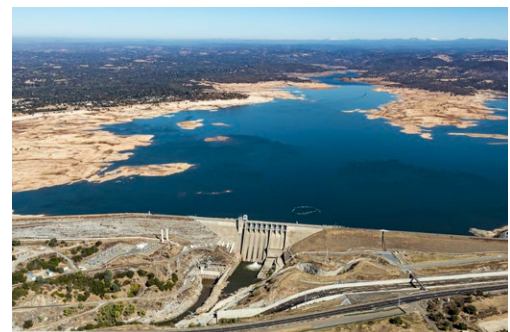
Aerial view of Folsom Dam in Sacramento County showing exposed banks. Photo taken October 28, 2021; courtesy of California Department of Water Resources
