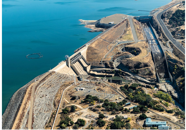
Photo of Folsom Dam and new auxiliary spillway in 2021.
