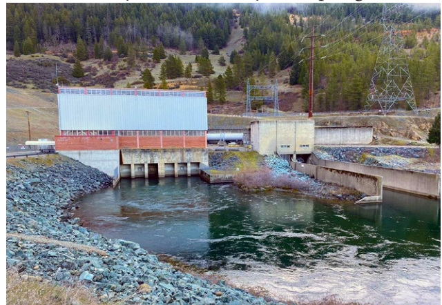
Trinity Powerplant at Trinity River has two generators with current total capacity of approximately 140 megawatts.
