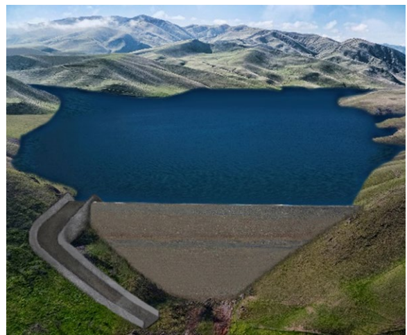
An artist’s rendering depicts the proposed Del Puerto Canyon Reservoir, a new offstream reservoir to develop more water storage south-of-the-Delta, received $15 million in 2022 funding for permitting, engineering, and design.
