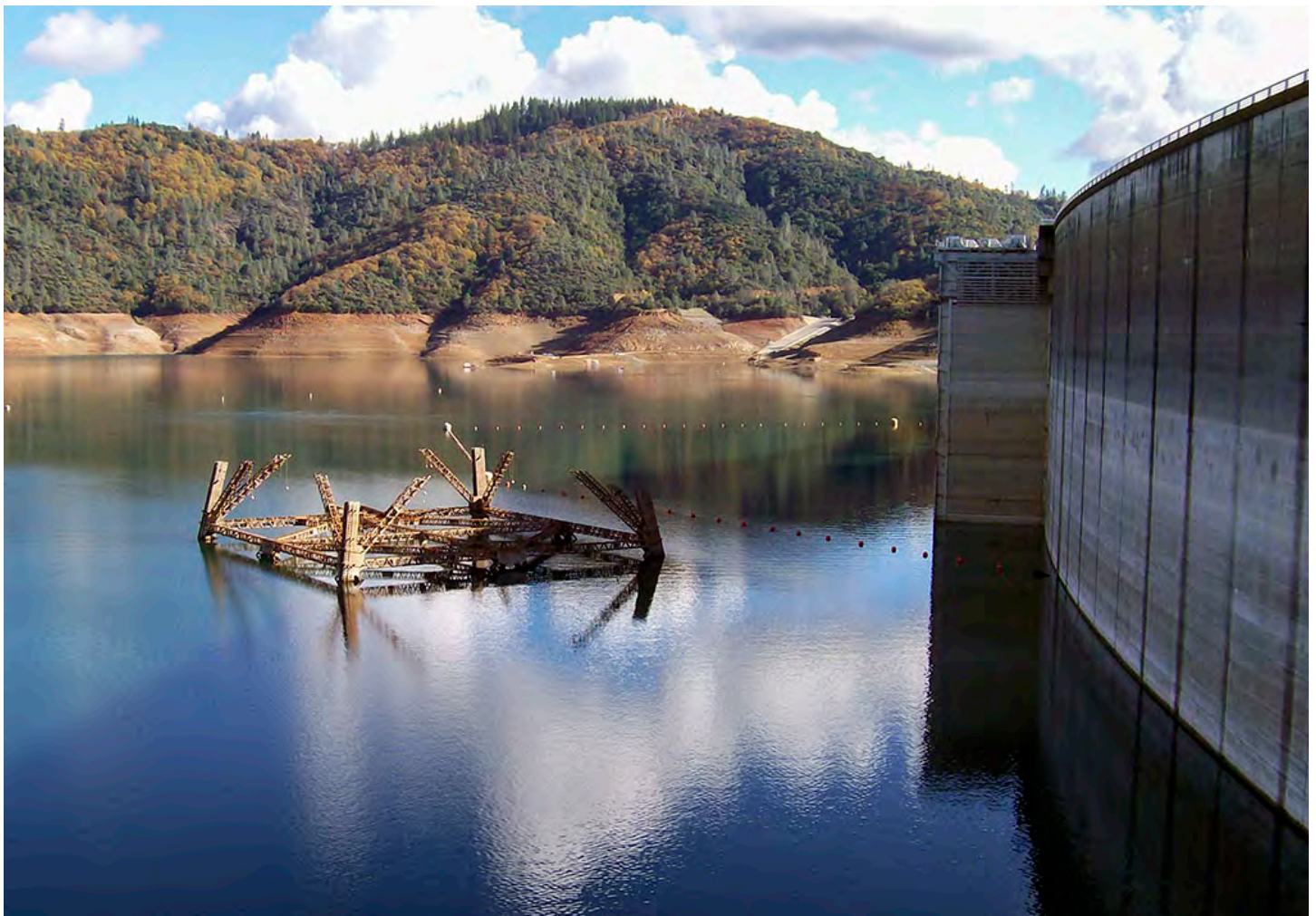
Temperature control device at Shasta Dam.
