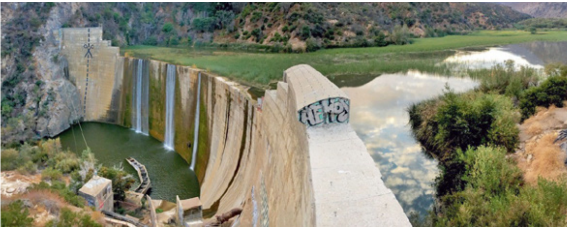
Matilija Dam in Ventura County, California (Surfrider Foundation/Paul Jenkin). Reservoir upstream of dam is transitioning to a wetland marsh and will eventually become riverine.
