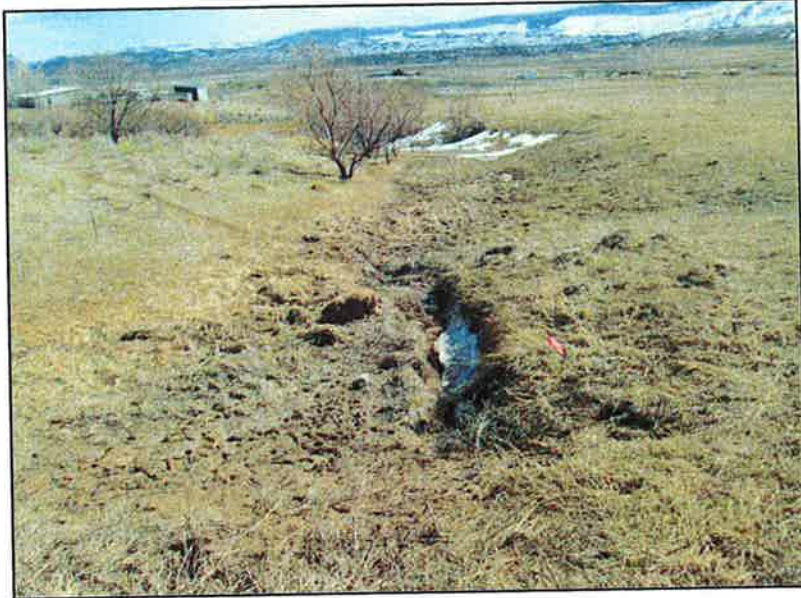
Photo 1: This photo illustrates the North West corner of the Habitat Replacement Site (HRS). An existing 6" overflow pipe, stemming from the stock/irrigation pond toward the north, enters the HRS at this location.
