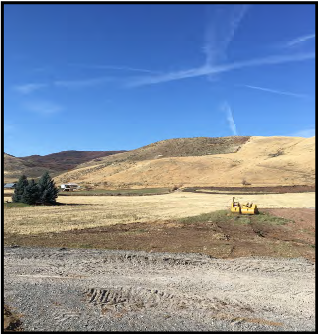
Second staging area along Morgan Valley Drive
