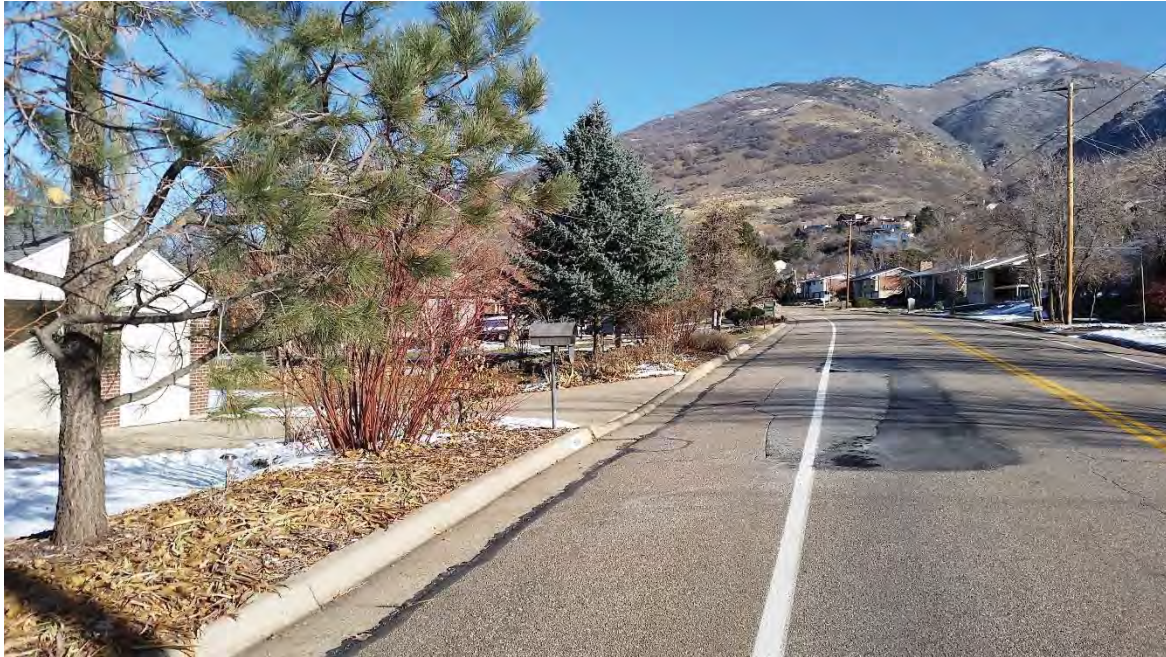
Figure 1. A typical residential street (Mountain Rd.) where buried pipe running along the shoulder would be replaced.
