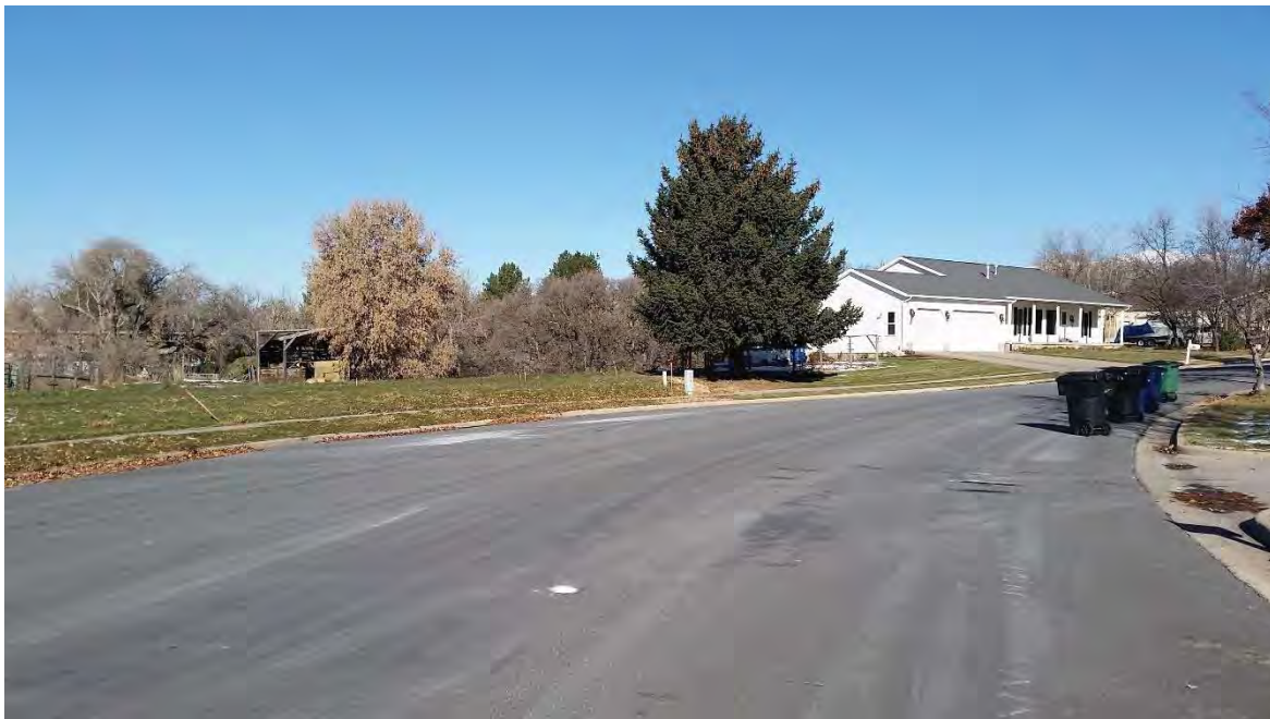
Figure 2. A typical residential street (Oak Ln.) where new pipe would be buried along the edge of the pavement.
