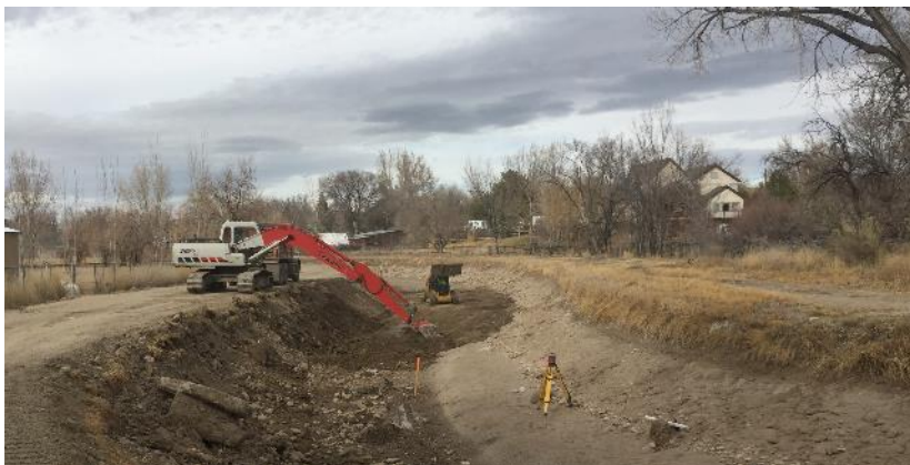
Machinery working to shape a canal in preparation for lining.
