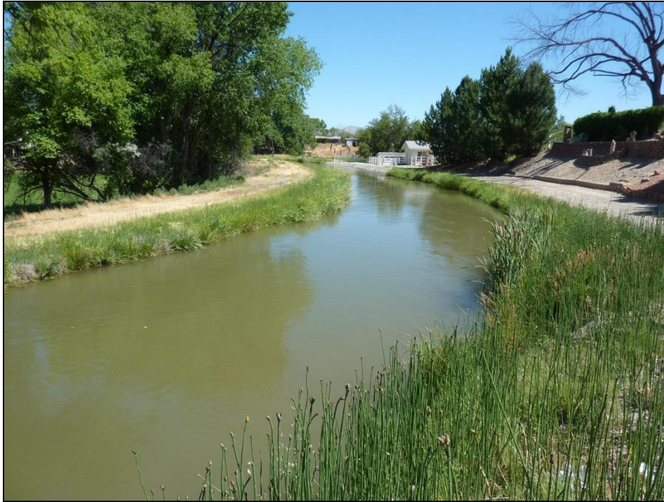
Photo 4. Section C of the Grand Valley Canal Lining Phase 4 -540 Project
