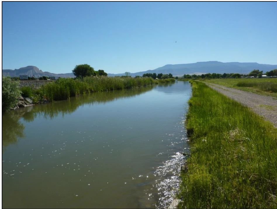
Photo 1. Section A of the Grand Valley Canal Lining Phase 4 -540 Project
