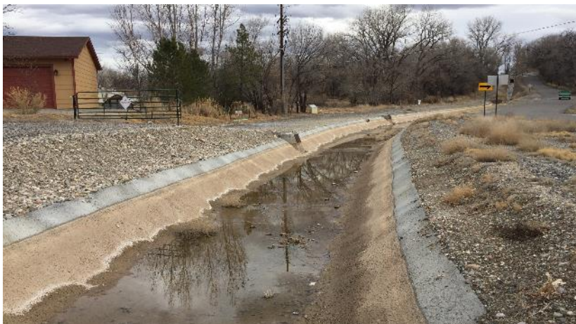
Example of a lined canal.
