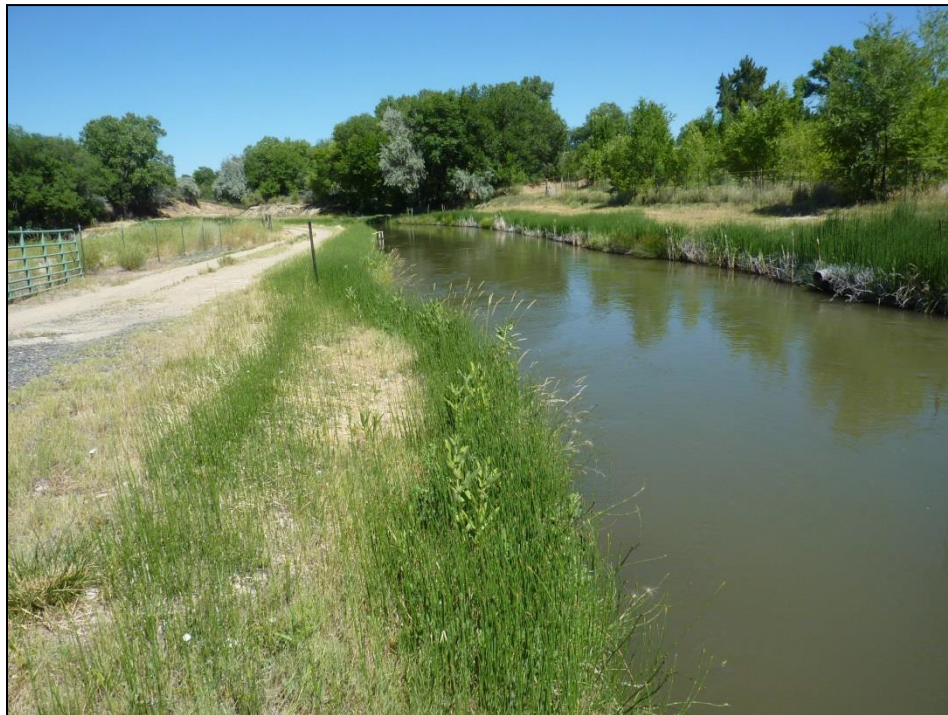
Photo 3. Section C of the Grand Valley Canal Lining Phase 4 -540 Project
