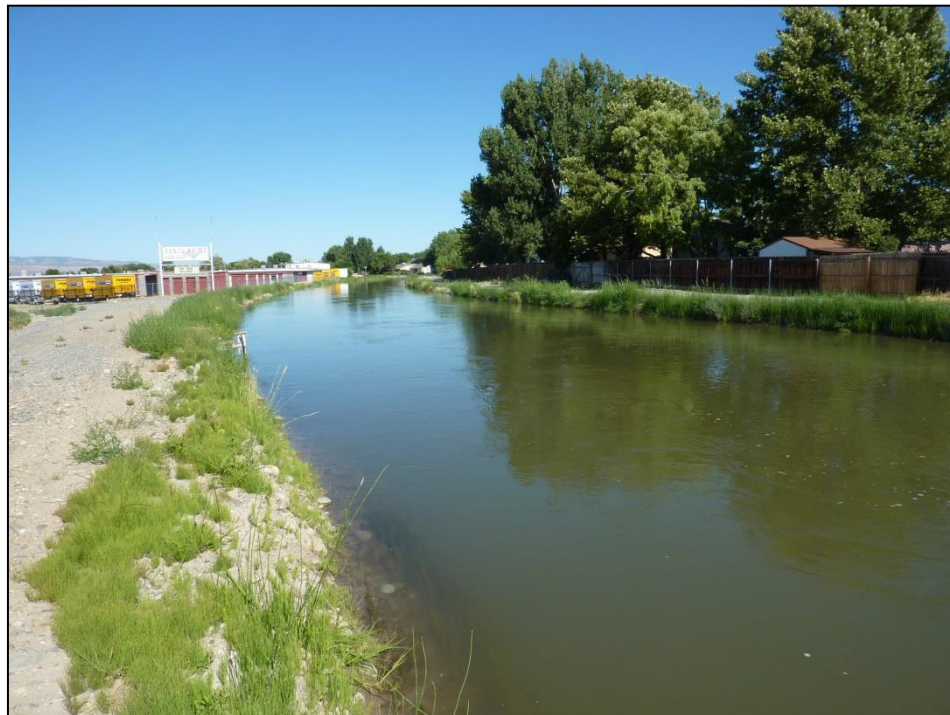
Photo 2. Section B of the Grand Valley Canal Lining Phase 4 -540 Project
