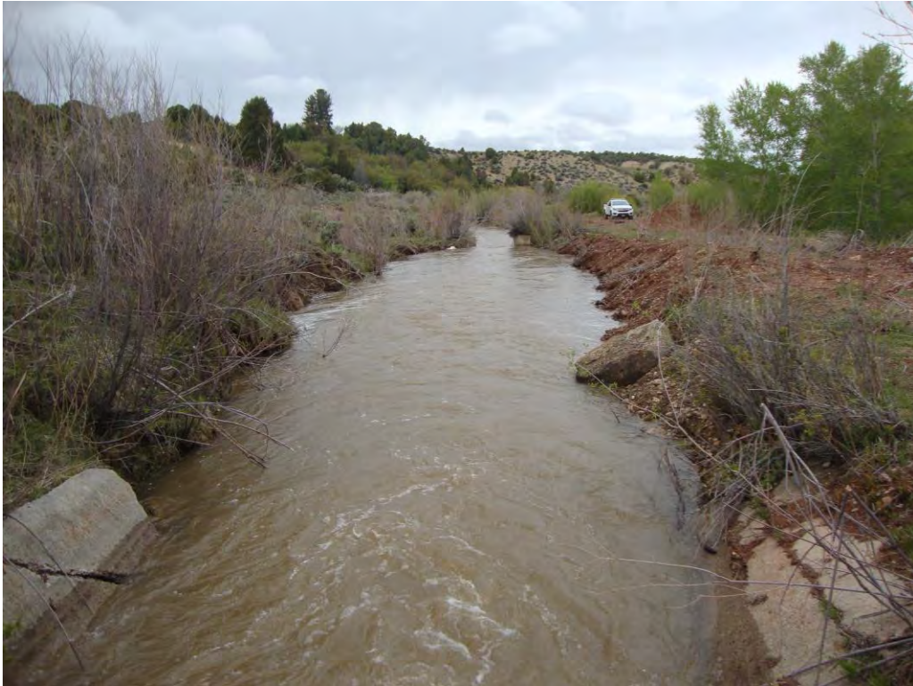
Photo 1. Start of Antelope Lateral, looking north and downstream from diversion structure.
