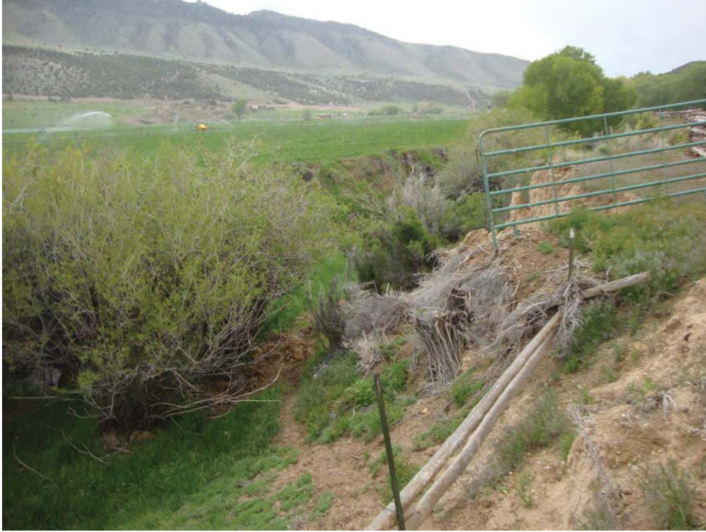
Photo 16. Segment N12, looking west.
