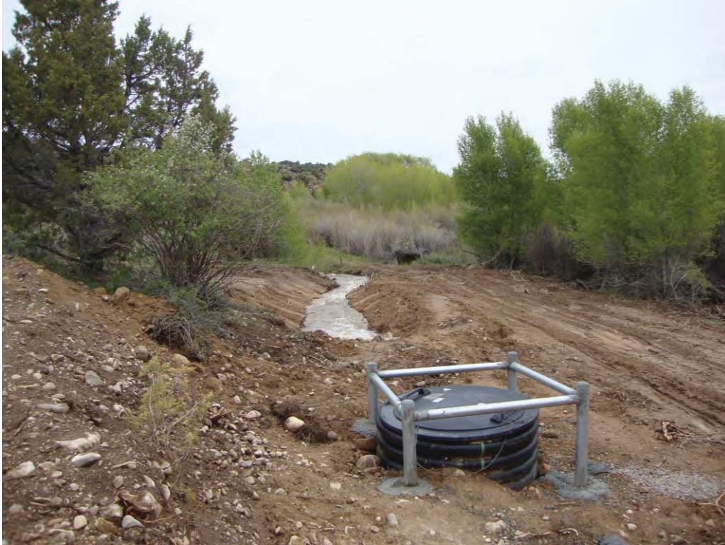
Photo 12. Segment N1 near diversion structure, looking northeast.
