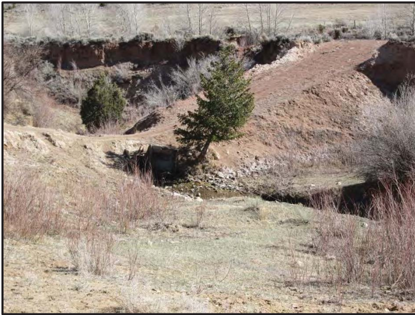
Photo 4: This photo shows an existing access road and location of the 4' CMP through which Birch Spring Creek flows (see the Habitat Replacement Site Exhibit).
