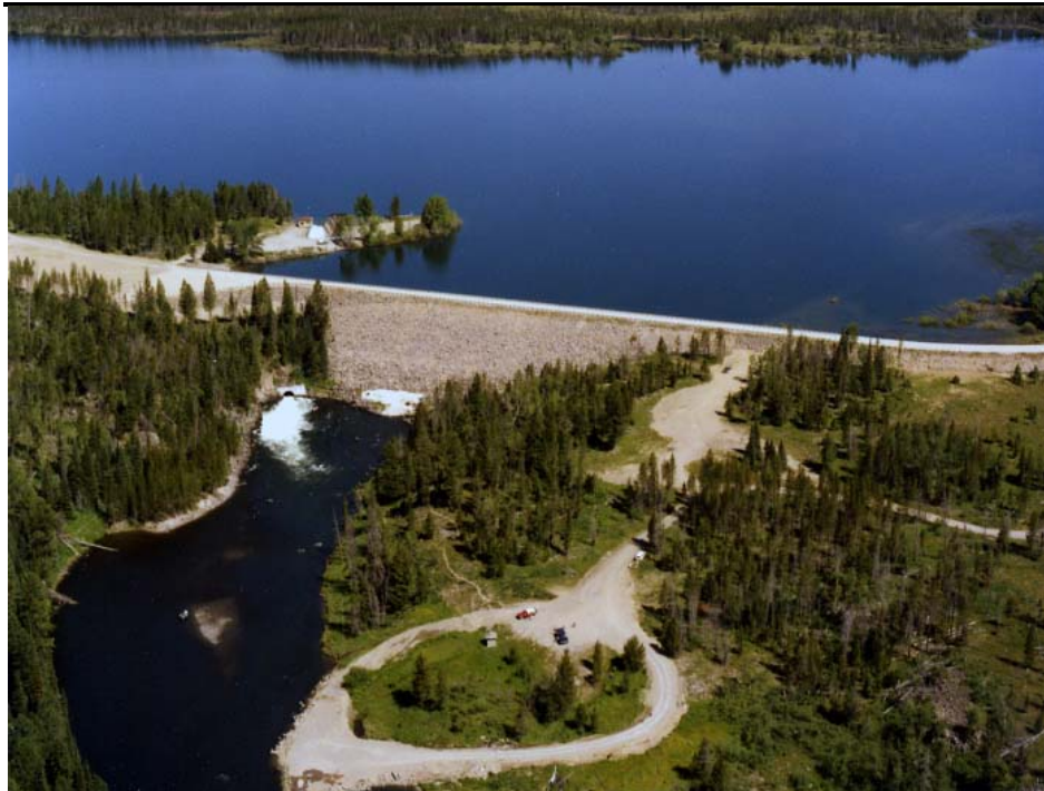
Figure 10. Island Park Dam and Reservoir on the Henrys Fork River, Idaho.
