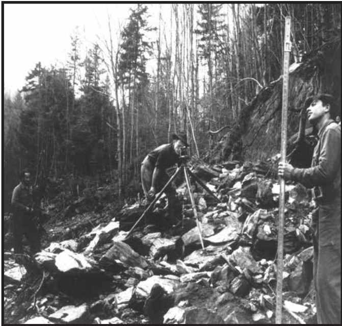
A CCC Crew working on road construction
