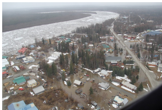
Fig 5: Photo of the flooding in McGrath, taken by a local pilot and accessed via the McGrath Community Message Board. Flooding impacted 15-20 residences as well as city infrastructure and roads.
