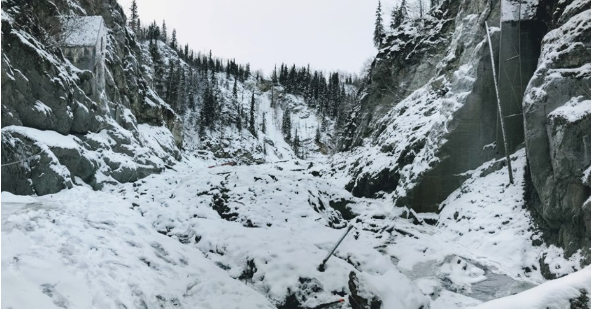
Photo: Looking upstream at remnants of the lower Eklutna Dam. Demolition of this concrete arch dam is ongoing. Credit: Crane Johnson, APRFC/NWS.
