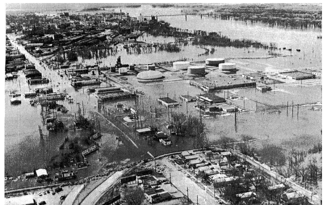
Photo: Flooding in La Crosse – Courtesy of La Crosse Tribune - April 1965
