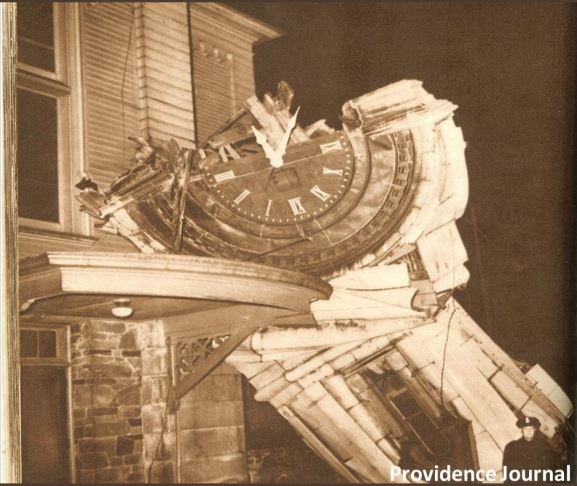
Above: Steeple from the Pawtucket Congregational Church was blown to the ground by the '38 Hurricane.
