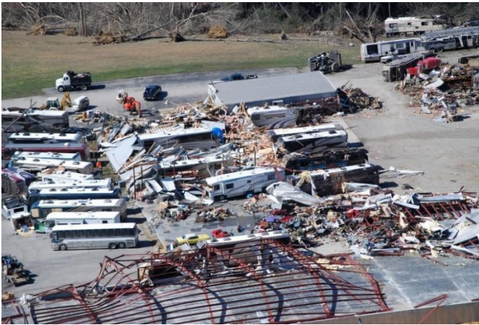
Aerial photo of damage in Laurel County
