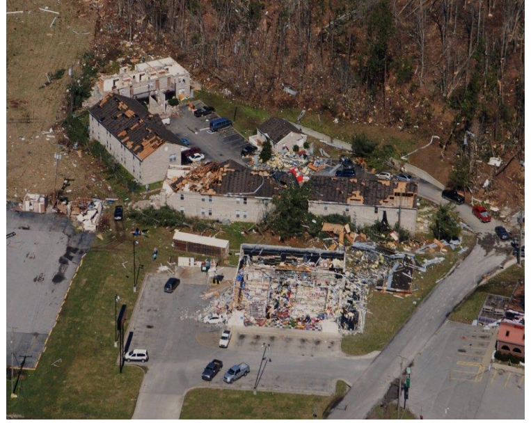
Damage to Salyersville in Magoffin County Courtesy of Allen Bolling
