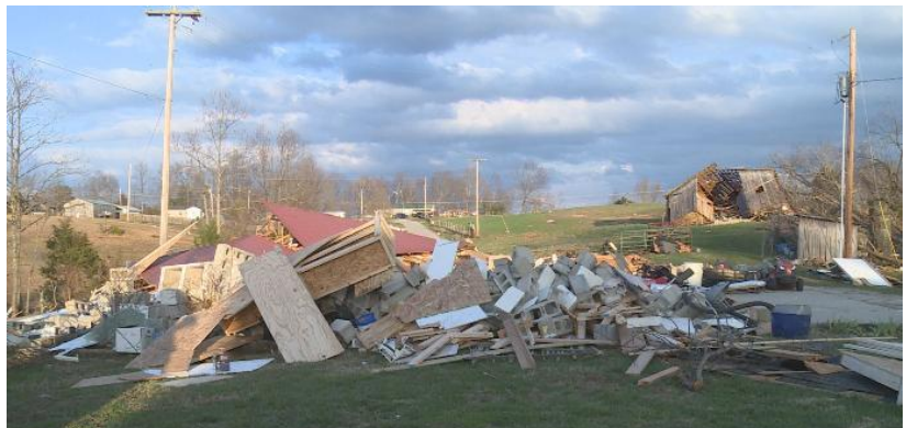
Structural damage at Winston in Estill County. Courtesy of WKYT
