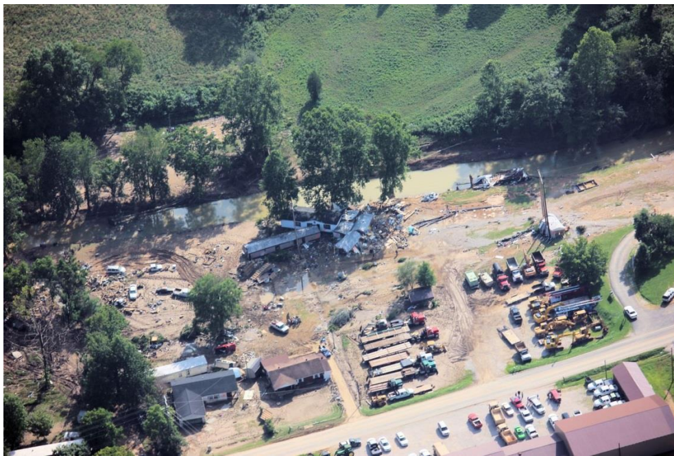
Post flood aerial photograph of damage along Highway 172. Photo courtesy of Randy Campbell, Huntington District, Corps of Engineers.
