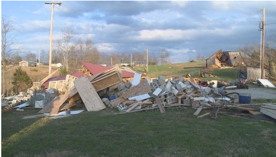
Wind damage in the Winston Community of Estill County. Courtesy of WKYT
