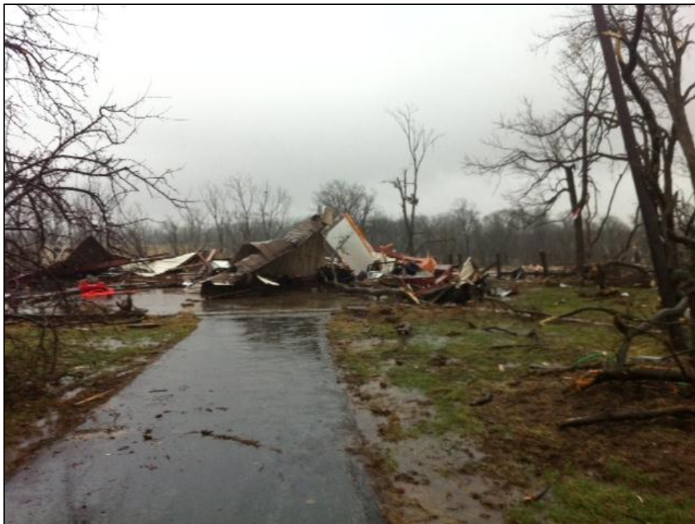
The picture to the left was taken by Kevin Harned of WAVE-3 news. It shows the complete demolition of a well - constructed barn.
