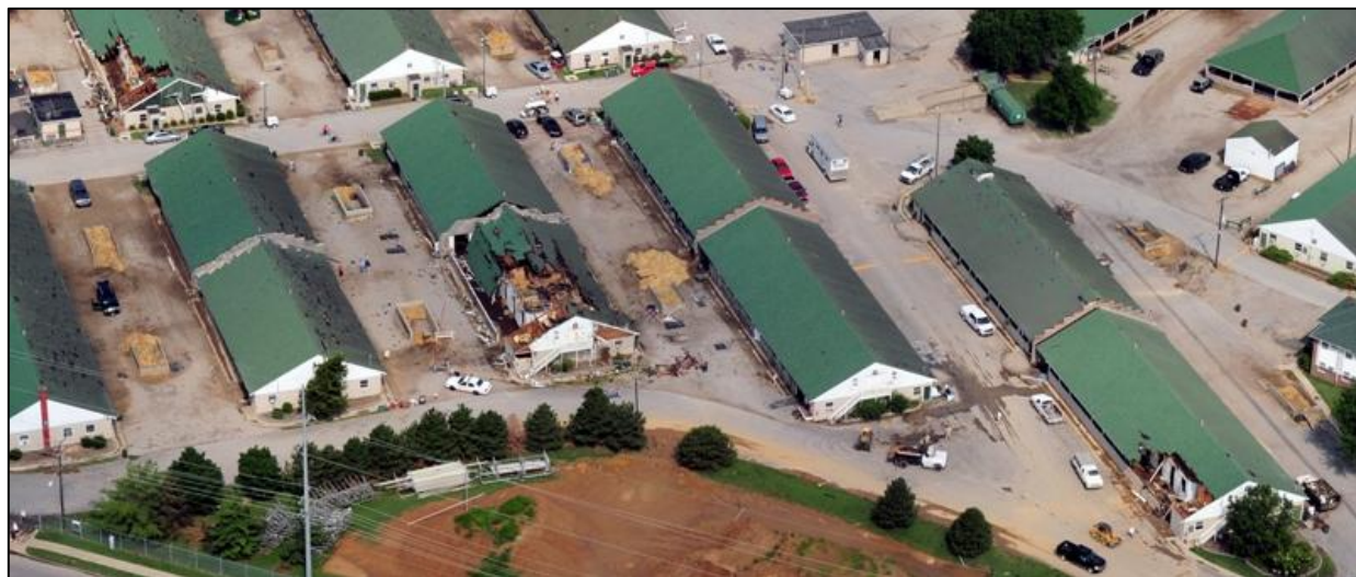
Damage to horse barns at Churchill Downs.
