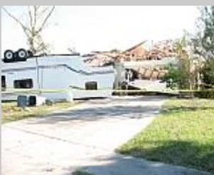
F1 damage to home in Seminole County
