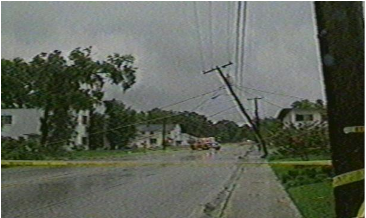
Power lines down
