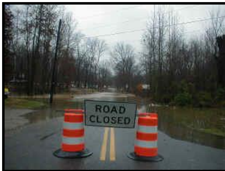
Road closed by flooding near Paducah, KY (photo by Shane Luecke)
